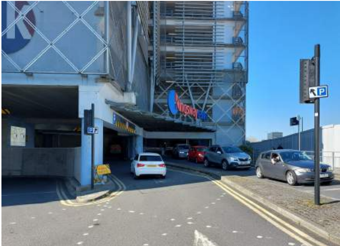
10. Looking North towards Kingsway Centre Parking Vehicle Entrance
