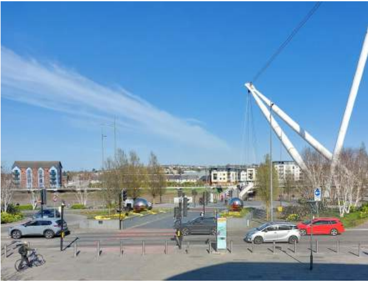
16. Looking North-East across Newport City Footbridge
