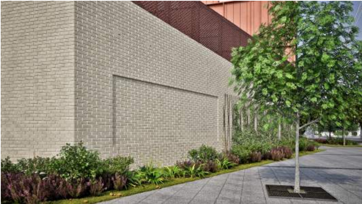
View of brickwork detailing - College logo in brick
