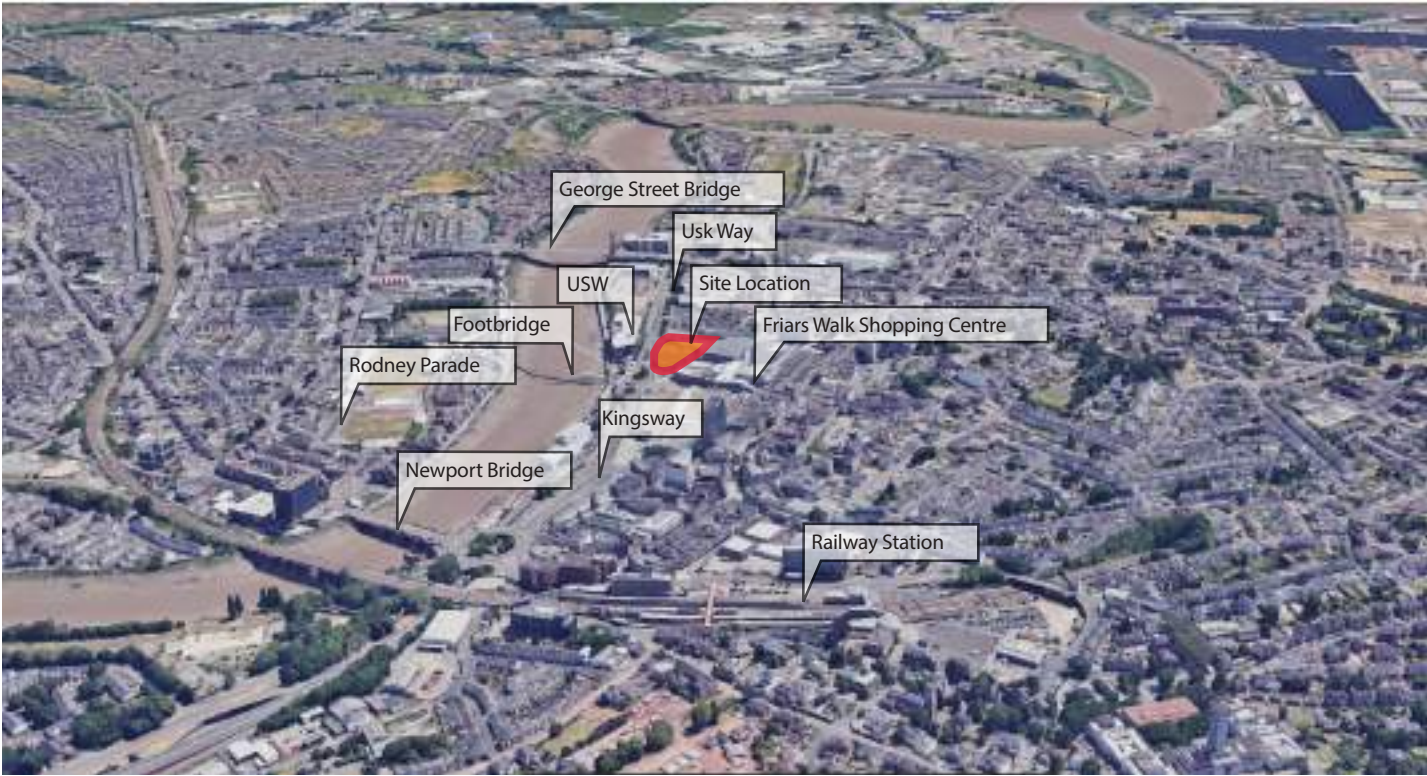
Google Earth Photo showing a bird view of Newport City
