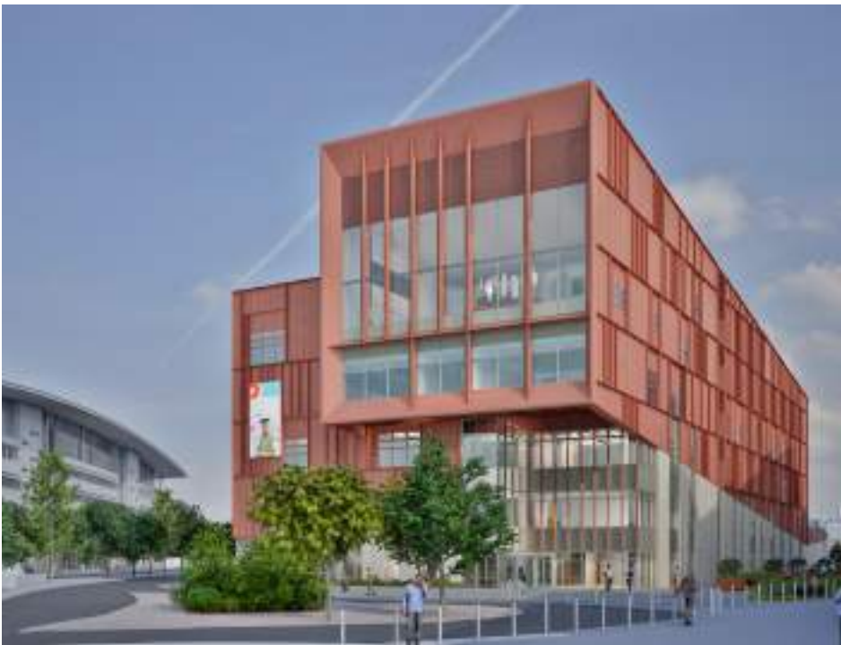
Render 2- The Entrance of the Building from the northwest (Usk Plaza)
