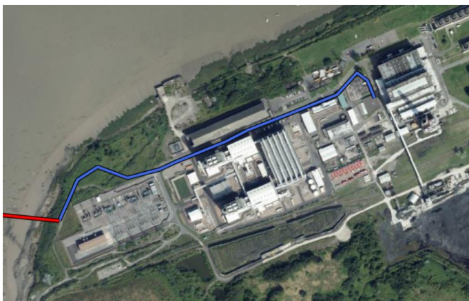
Figure 2.1 Uskmouth Power Station. Air photo source: Bing Maps (not to scale).
