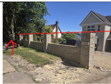
Before 'oyster white' fencing infill panels and solid similar gates are in place as indicated by the red line
