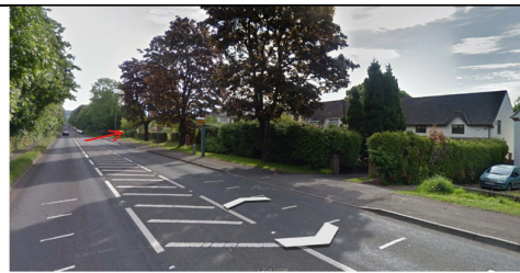
Chepstow Road looking east
