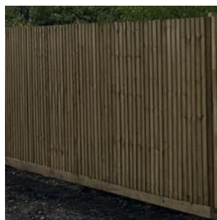
Existing Boundary Fence Close Boarded Timber Fence
