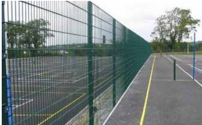
Proposed 2.4m weldmesh perimeter fencing
