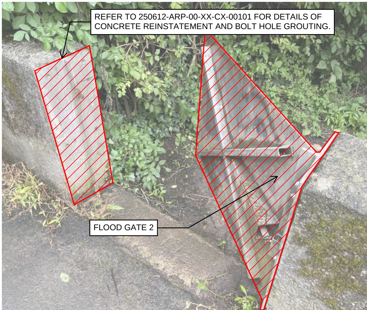
PHOTO 2: FLOOD GATE 2 (NTS)
