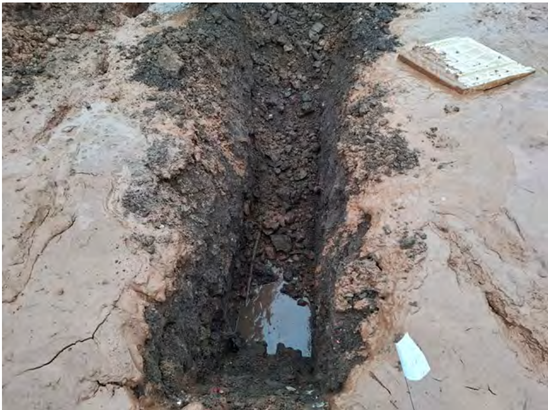
Trial Pit TP09 – Excavation
