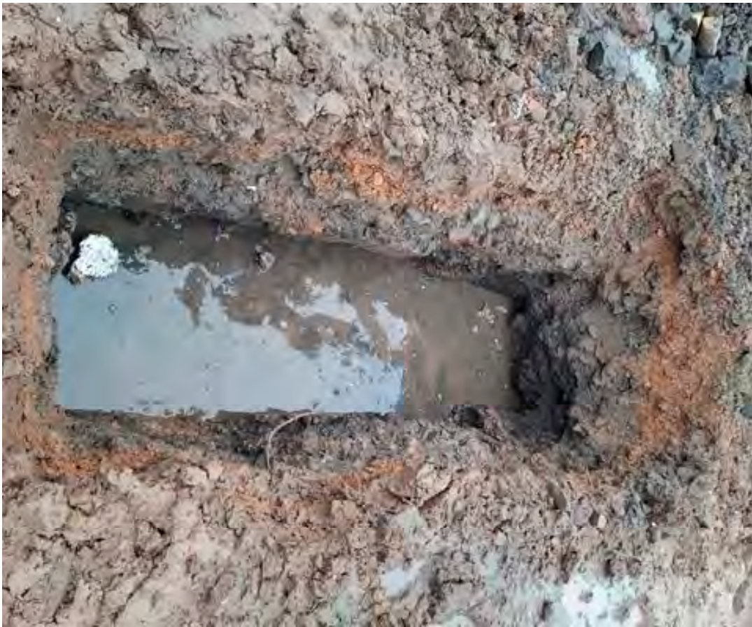
Trial Pit TP01 – Pit and groundwater level
