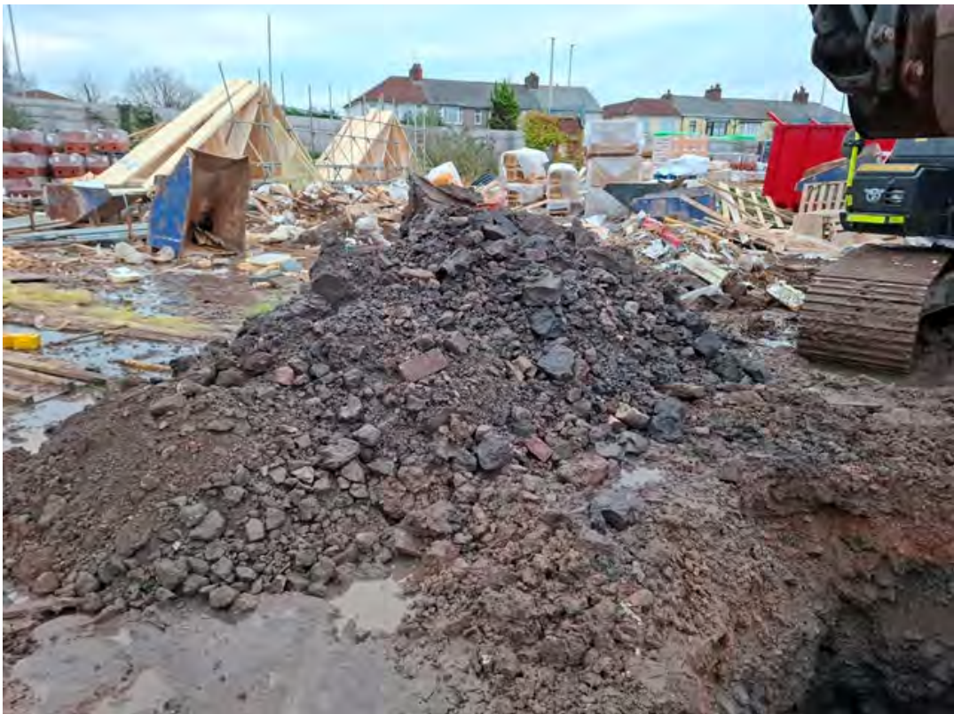
Trial Pit TP01 – Made Ground arising
