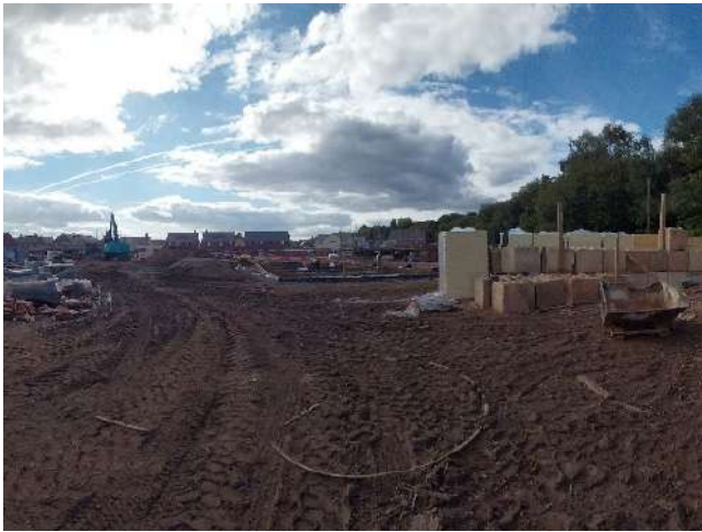
Photograph 1: Overall view of the site, looking north-west.
