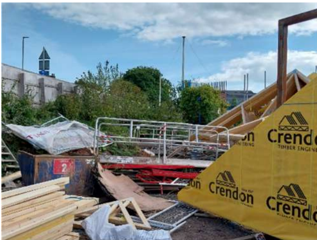
Photograph 3: South-east direction of the restricted access zone in the north/eastern section of the site.
