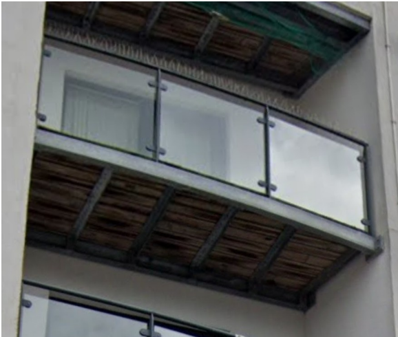
Existing timber balconies
