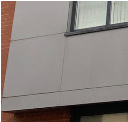
Existing HPL Cladding
