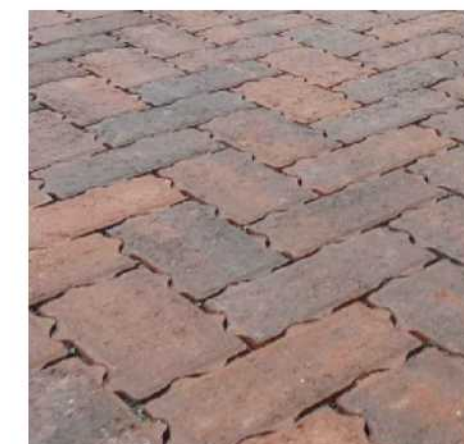
PERMEABLE BLOCK PAVING
