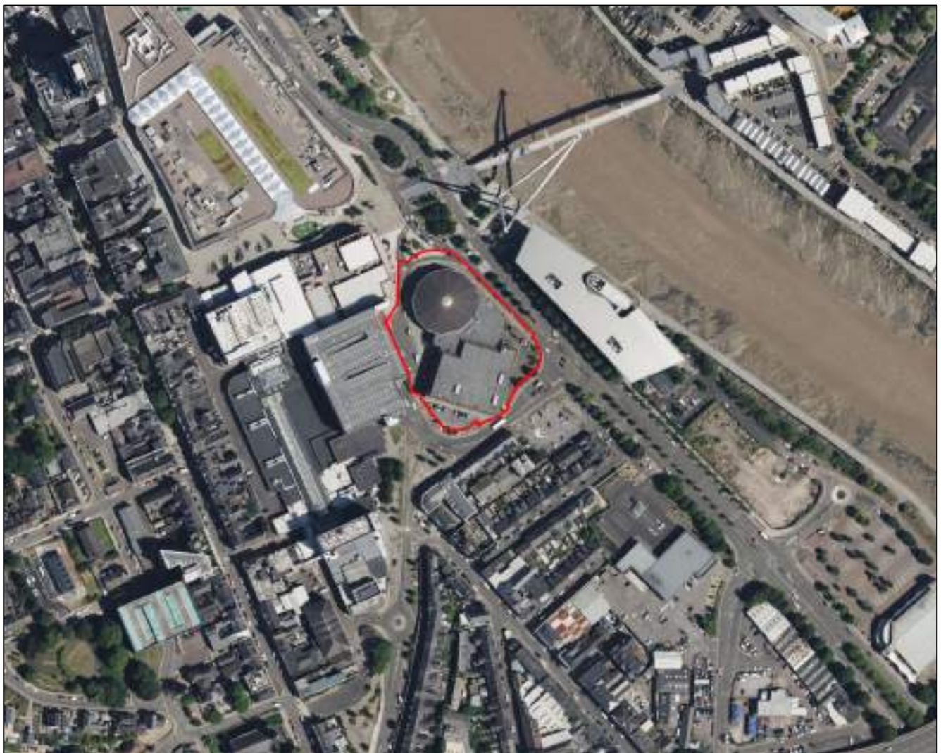
Figure 2-2. Satellite Visual of Site (pre-demolition, accessed 16th June 2026)
