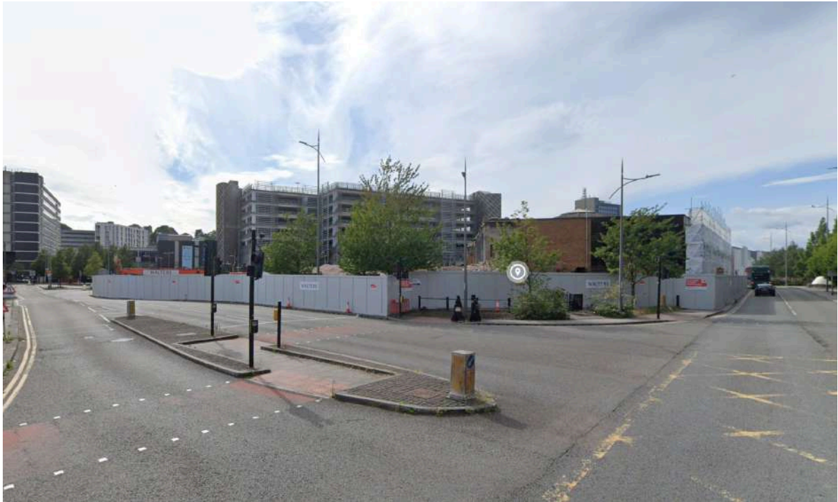
Figure 3: View from the South-east (Kingsway Multi-Storey Car Park across).
