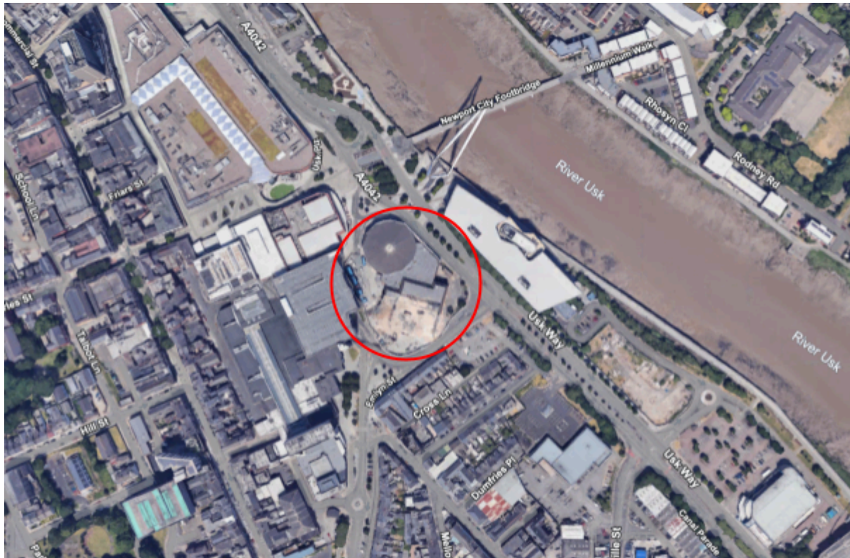
Figure 3: Aerial Photograph of Site - Approximately defined by the Red Circle, with the former Leisure Centre now demolished still shown.
