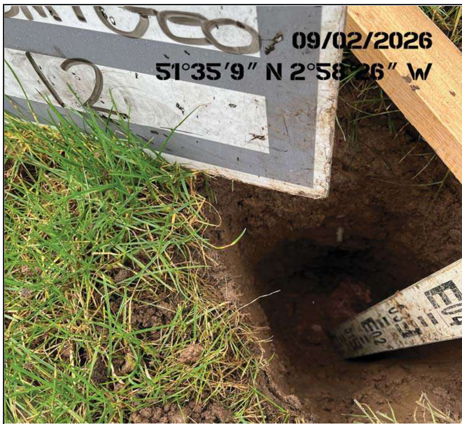
Plot 12 Trial Pit Membrane Placement
