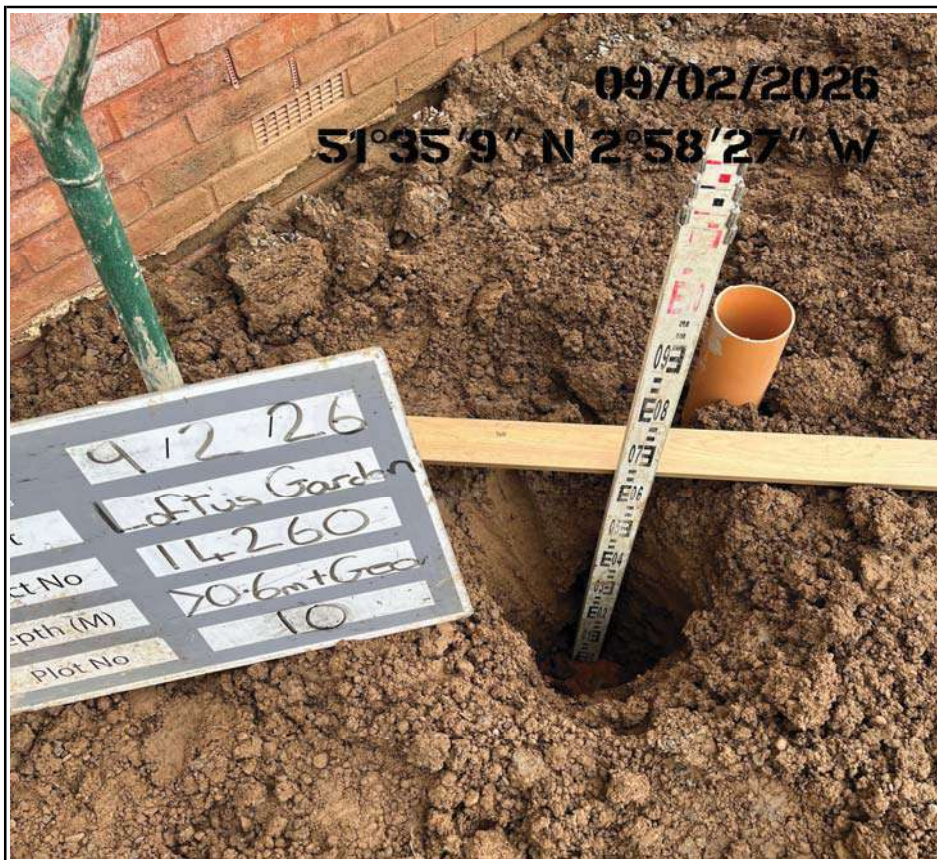
Plot 10 Front Garden Trial Pit Capping Depth Check
