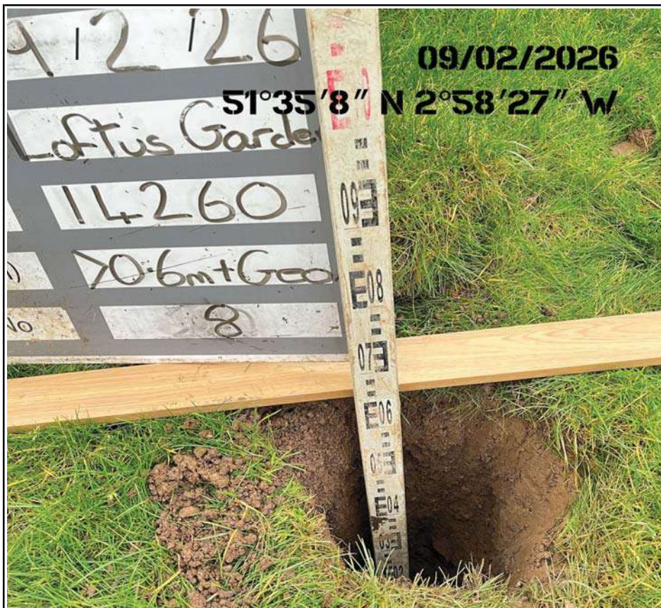
Plot 8 Trial Pit Excavation
