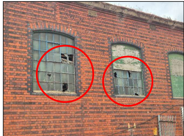
Figure 11 – Damage to Windows on (NE) Wall of Shed 4, Offers Potential Access/Egress for both Crevice and Void-Dwelling Bats to Shed 4 Interior via these Areas
