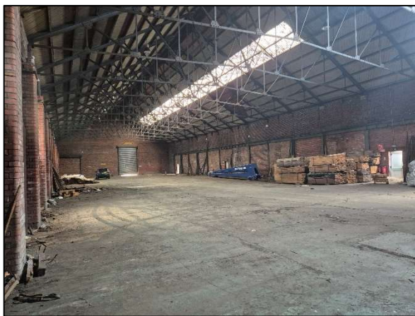
Figure 12 – Shed 4 Interior, Looking (SE)
