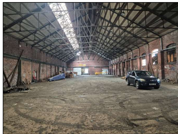
Figure 13 – Shed 4 Interior, Looking (NW)
