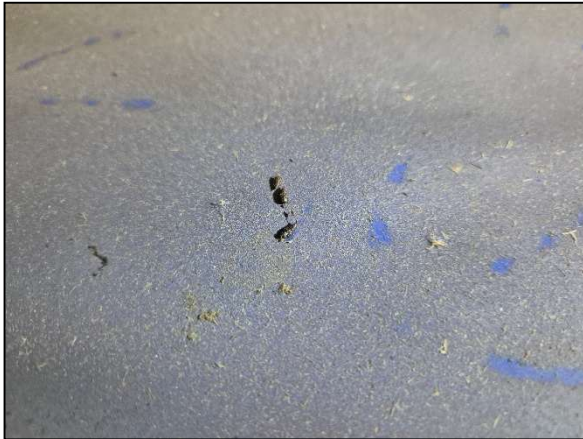
Figure 22 – Bat Droppings on Equipment in Shed 4
