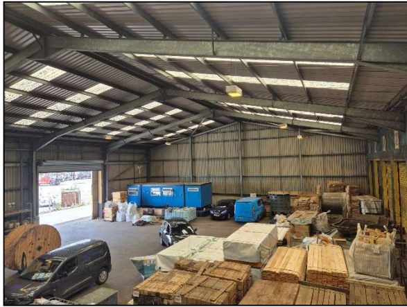
Figure 20 – GF Stores. Interior, Looking (SE)
