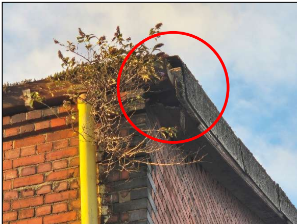
Figure 10 – Damage to Timber Soffit on (SW) Corner of Shed 4, May Offer Potential Roosting Opportunity for Crevice-Dwelling Bats
