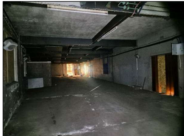
Figure 19 – Interior of Ground Floor of Affixed Brick Building at (E) Side of MSB. The Room is Dark and Cooler than the Main Warehouse Building.
