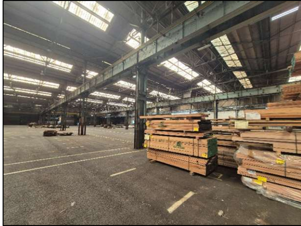
Figure 16 – Neptune Works Interior, Looking (SW)
