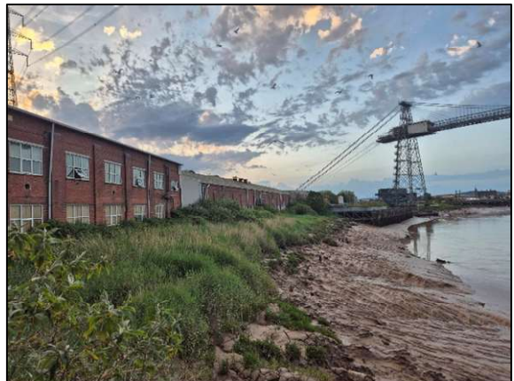
Figure 12 – Additional view of (E) Side of MSB
