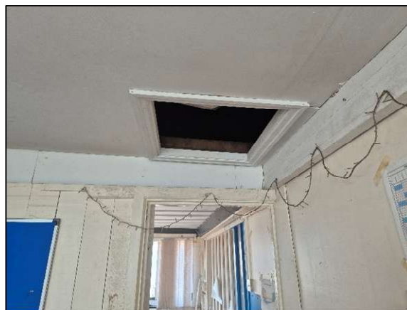
Figure 25 – Loft Hatch at 1 st Floor Level within Kitchen at (S) End of Brick Building
