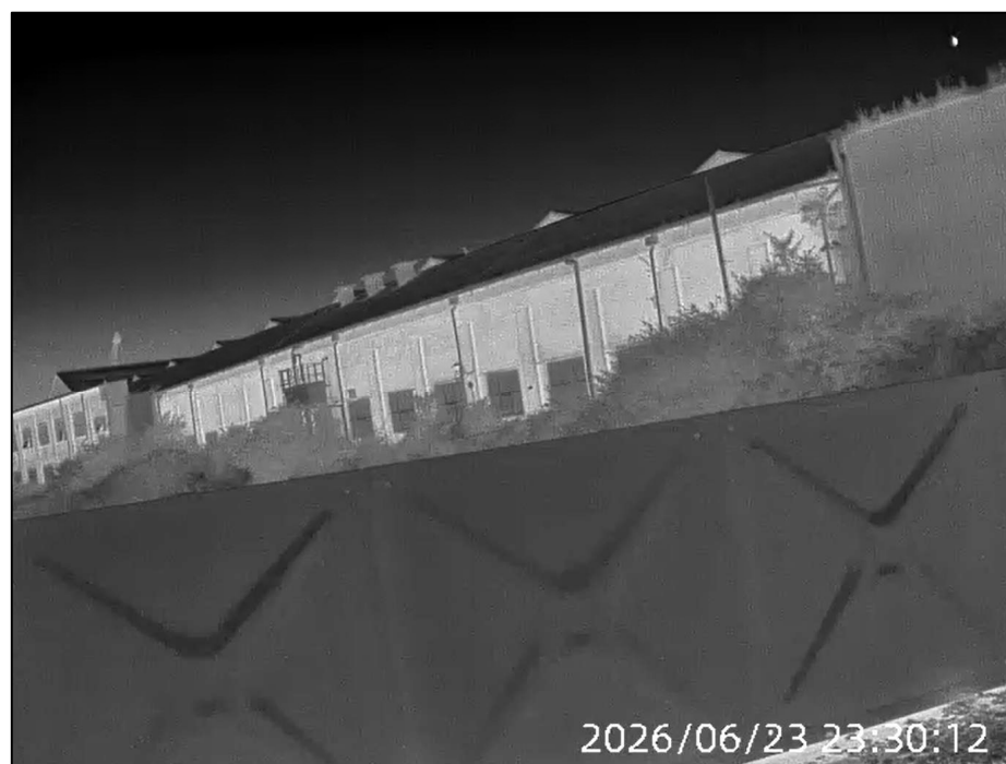
Figure 30 – Thermal Imaging of (E) Aspect of Neptune Works Warehouses
