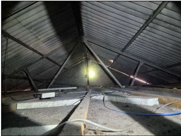
Figure 26 – Interior of Loft of at (S) End of Brick Building. Exposed Steel Framework visible, suitable for Free-Hanging Bats
