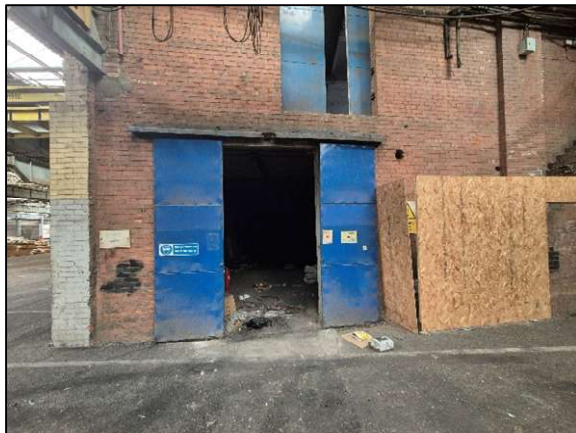
Figure 18 – Access Point to Ground Floor of Affixed Brick Building at (E) Side of MSB via Open Double-Doors
