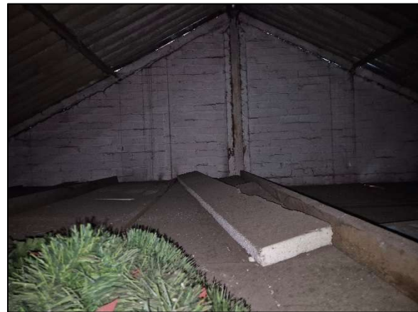
Figure 27 – Brick Wall at (S) End of Loft Interior. Brickwork in Generally Good Condition, Reducing Potential for Crevice-Dwellers
