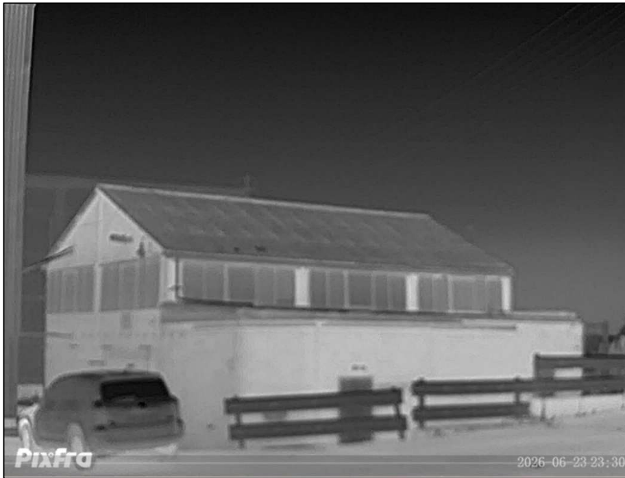
Figure 33 – Thermal Imaging of Brick Building at (S) of Neptune Works Warehouses
