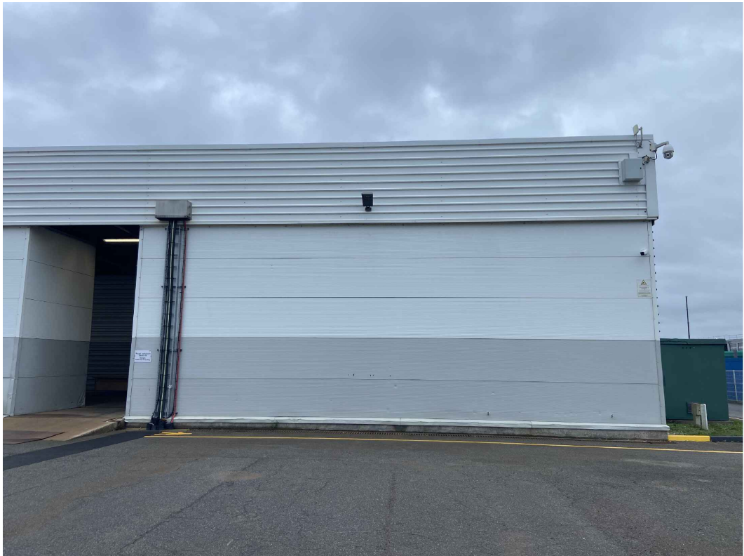
EXTERNAL ELEVATION OF GENERATOR ROOM
