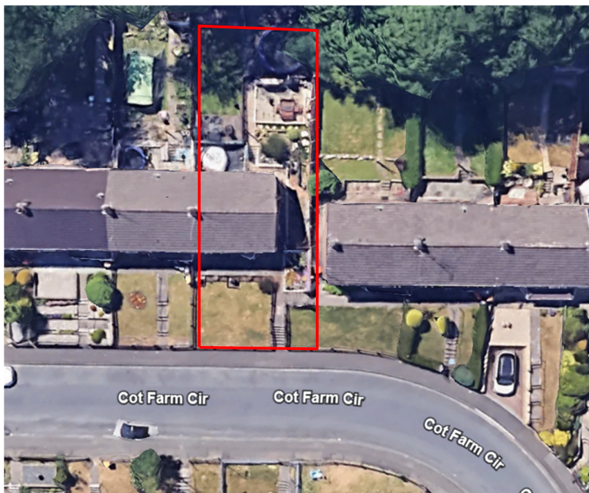
Figure 1: 21 Cot Farm Circle and surrounding properties.
