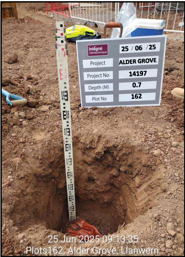
Plot 162 Capping Validation Depth Check
