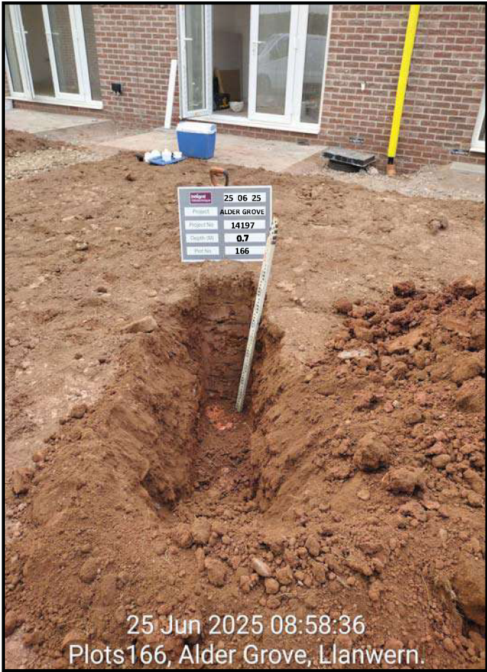
Plot 166 Capping Validation Depth Check
