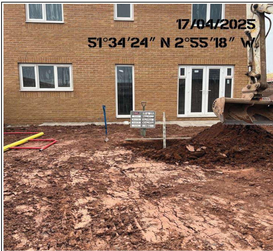
Plot 180 Capping validation Depth Check
