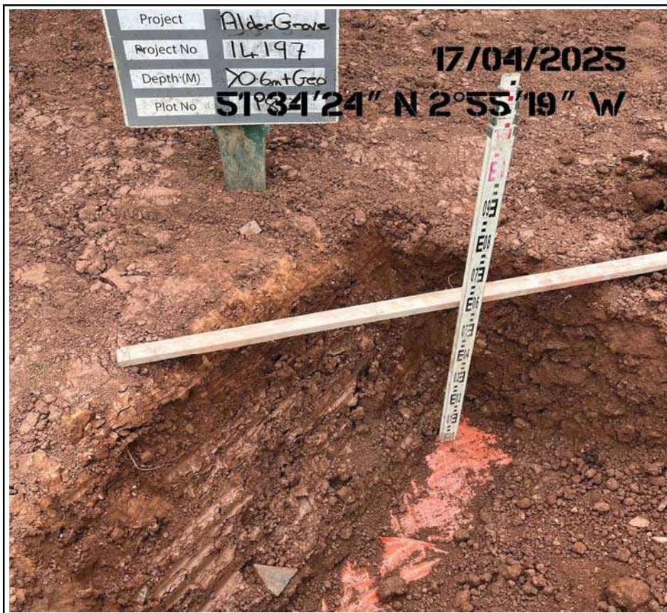
Plot 180 Membrane Placement
