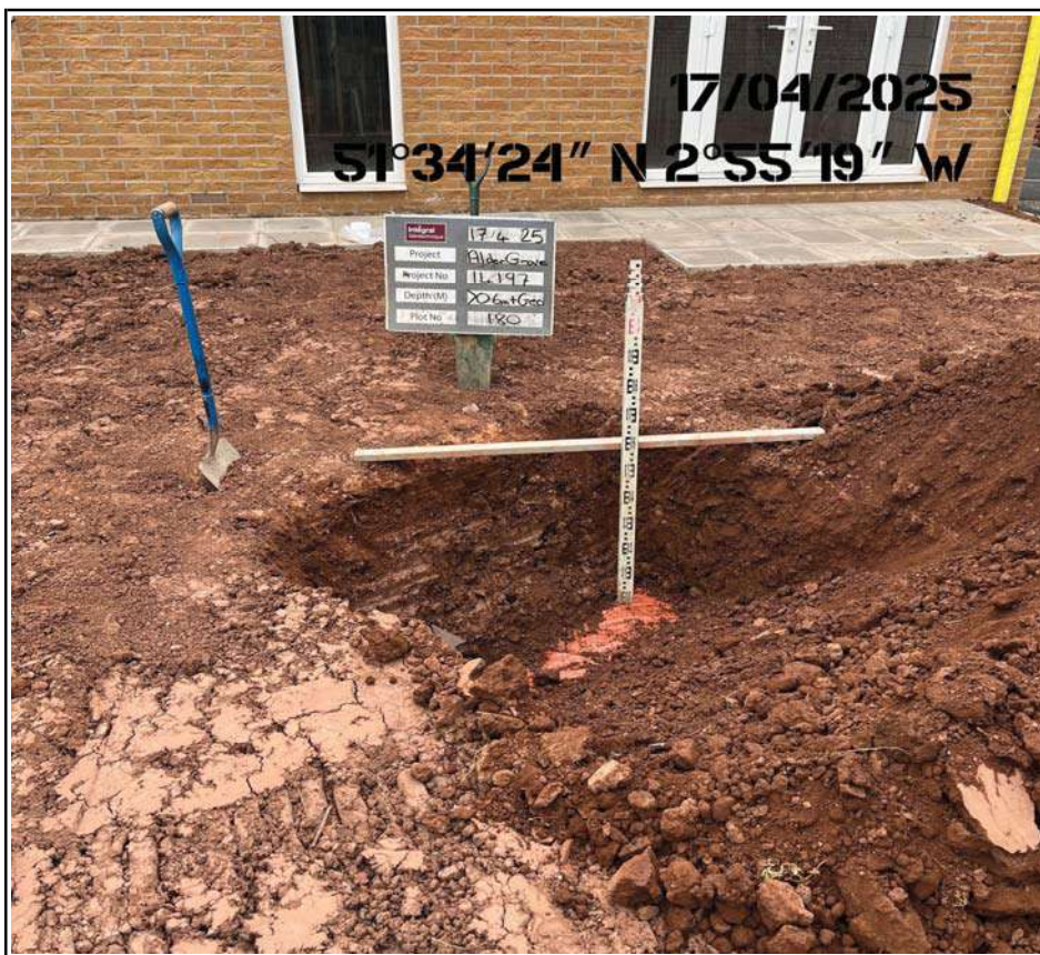
Plot 180 Trial Pit Excavation Profile
