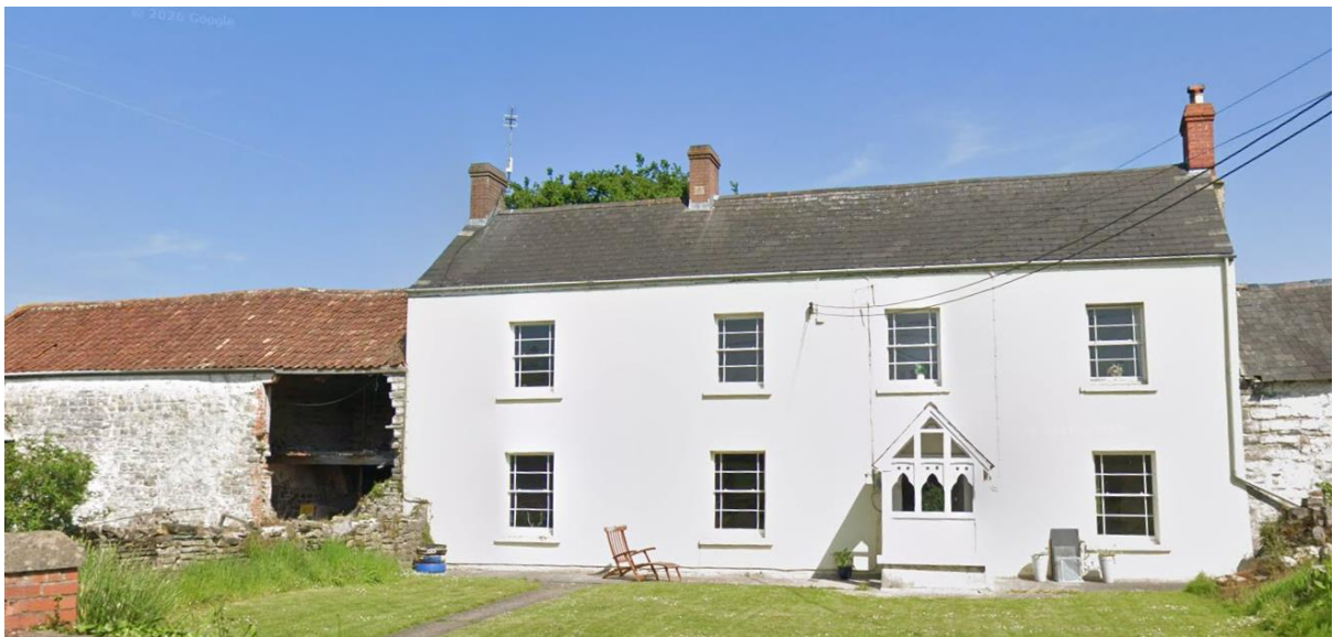
Figure 12: Samson Court, western elevation, May 2025.
