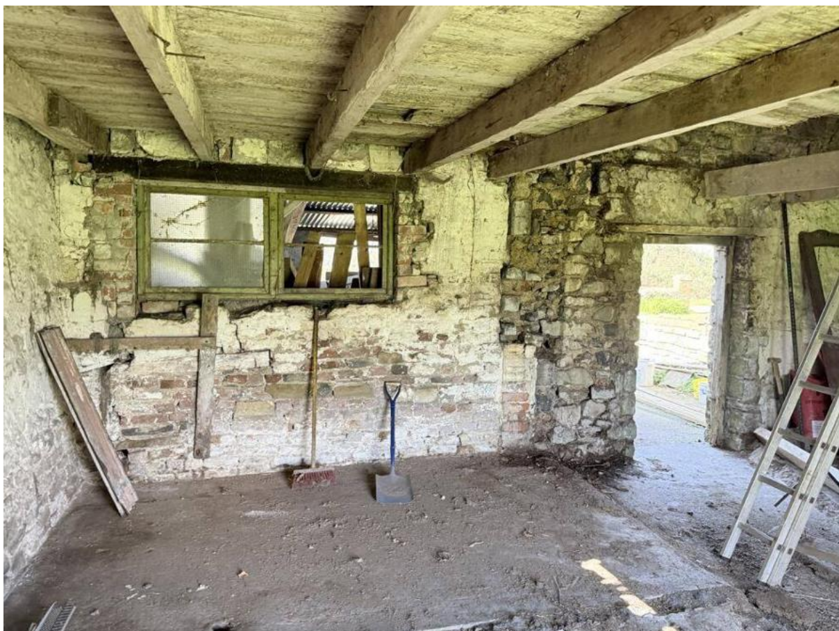
Figure 13: Interior of the asset showing historic floorboarding in situ, March 2026
