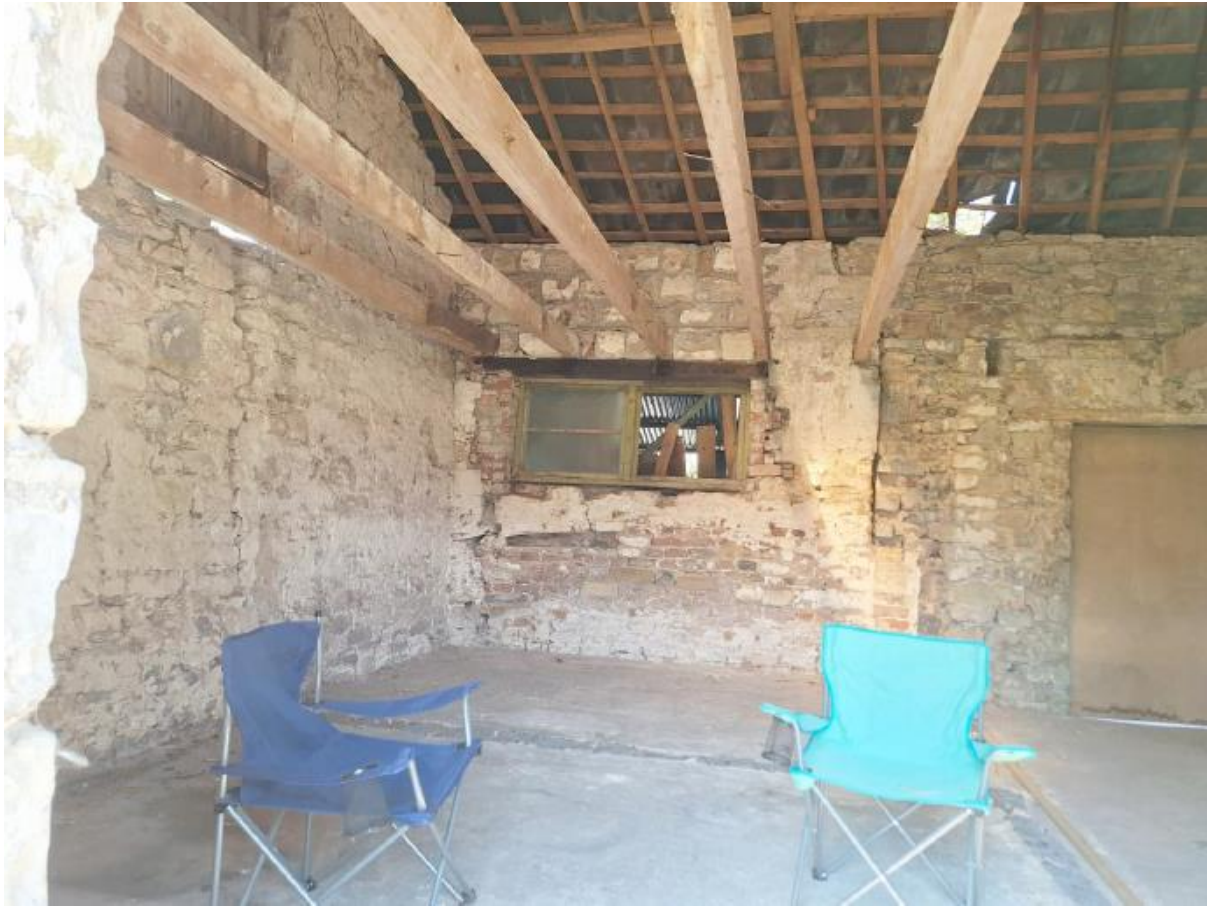
Figure 14: Interior of the asset showing historic floorboarding removed, July 2026
