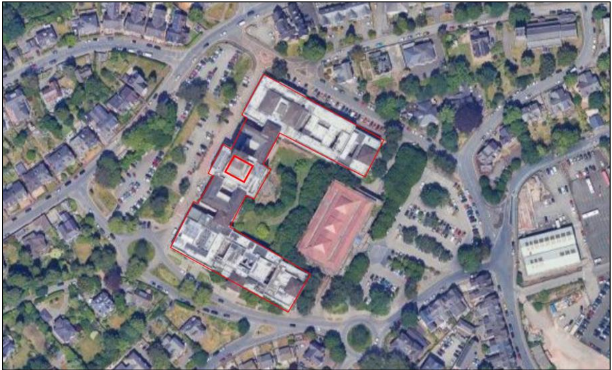
Figure 3-1 – Site Location Arial view
