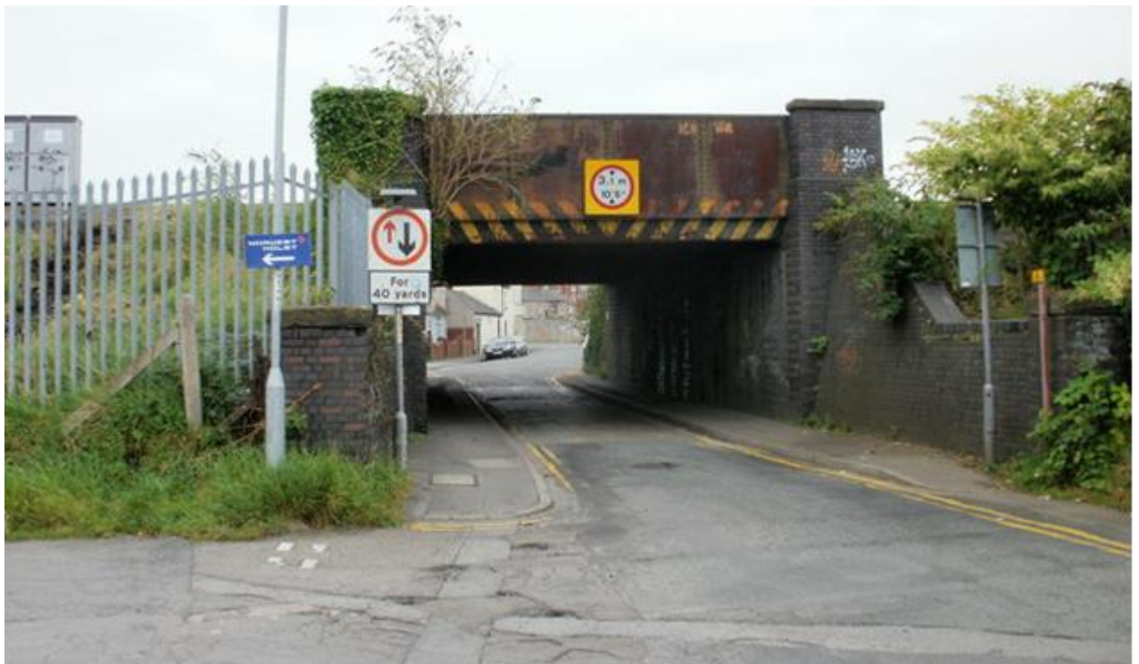
Image of 3.1m height restriction on Route A
