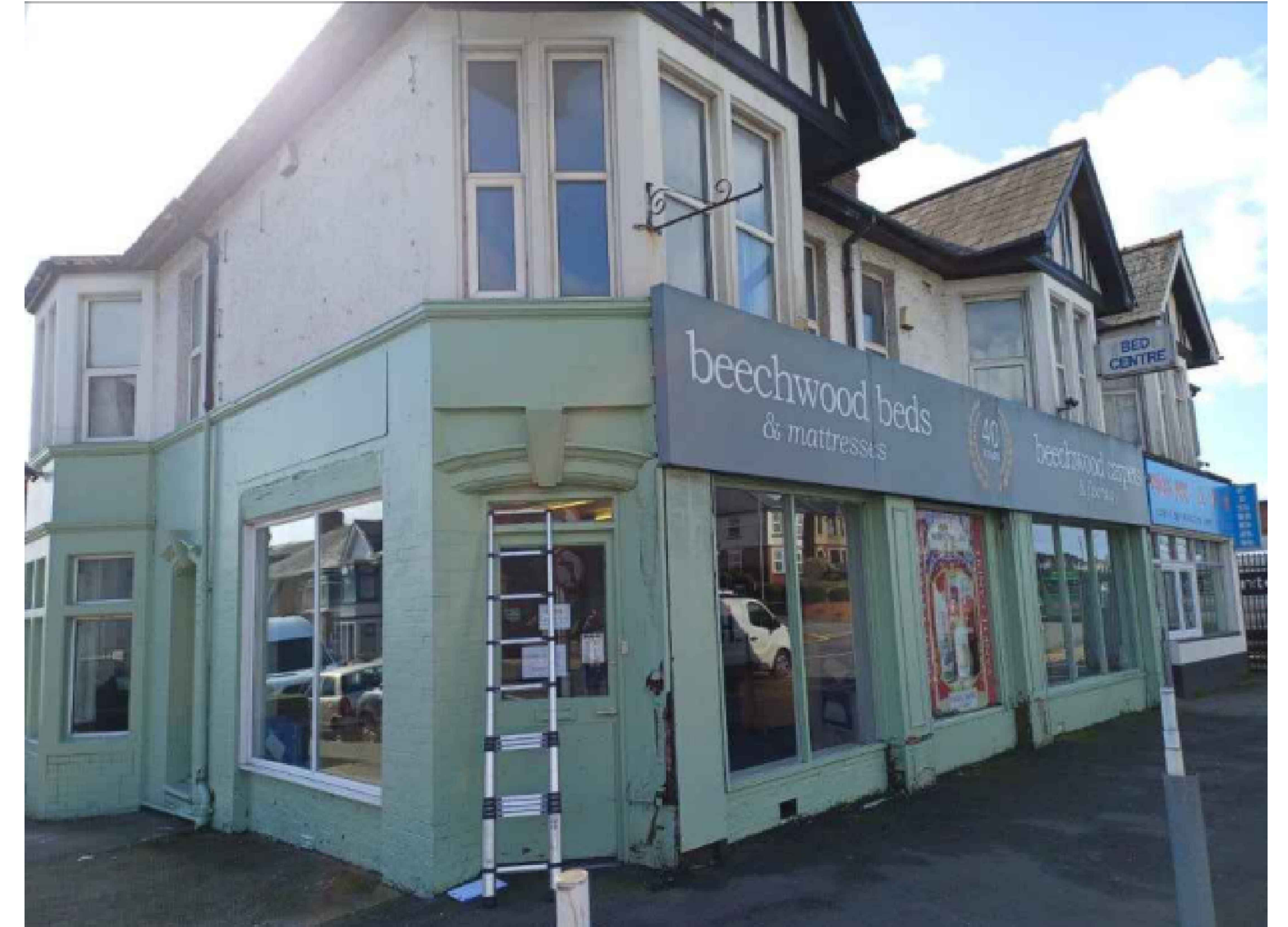
PHOTO OF EXISTING FRONT ELEVATION
