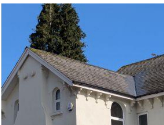
The roof was well-maintained with minor sections of raise tiles and lead flashing.
