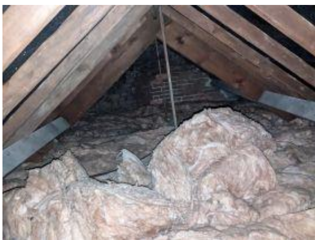
Internal - PRFs – Cavity above bitumen membrane.
