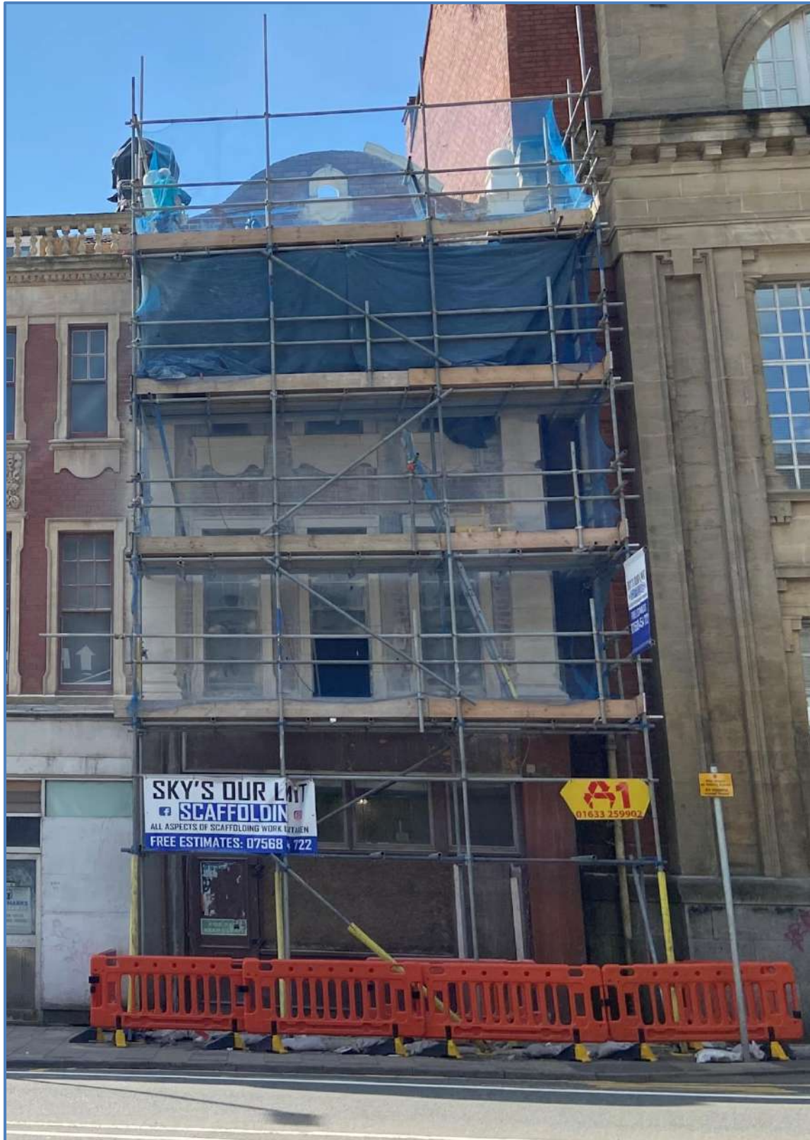
Image 1 – Front elevation of. No.10 Clarence Place, during current repair works to masonry.
