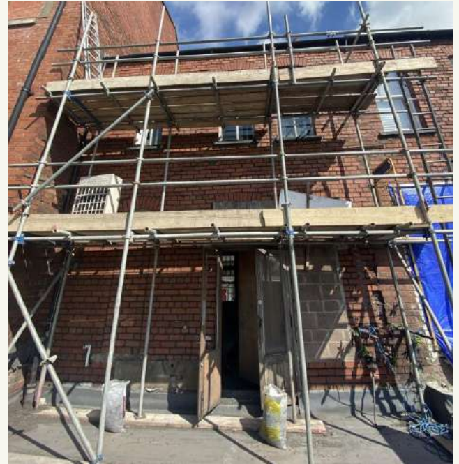
Figure 3.10 – Rear elevation of no.10, photo taken during recent repair works (March to June 2021).
