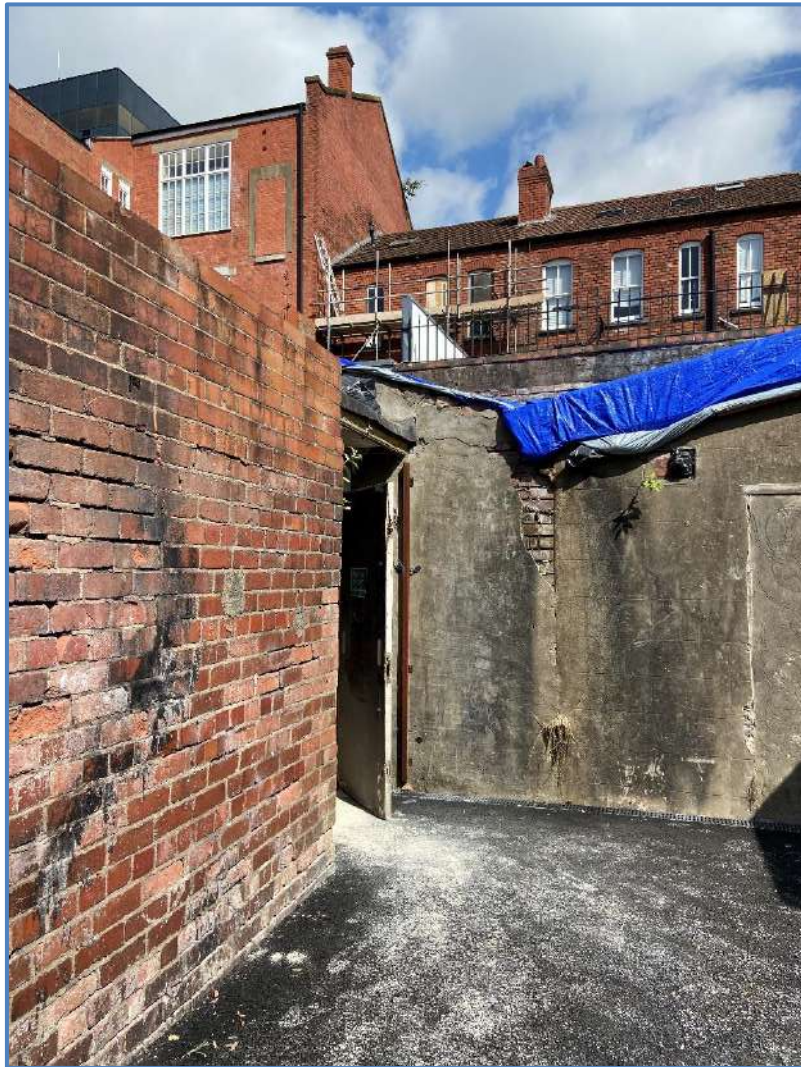
Images 5 and 6 – Rear elevation of no.10 Clarence Place.
