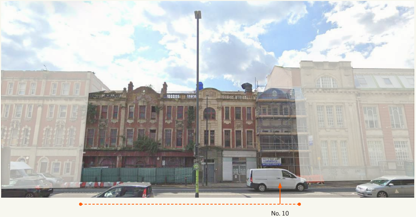
Figure 3.1 – From left to right: 20-34 Clarence Place, 10-28 Clarence Place and the Technical Institute.
