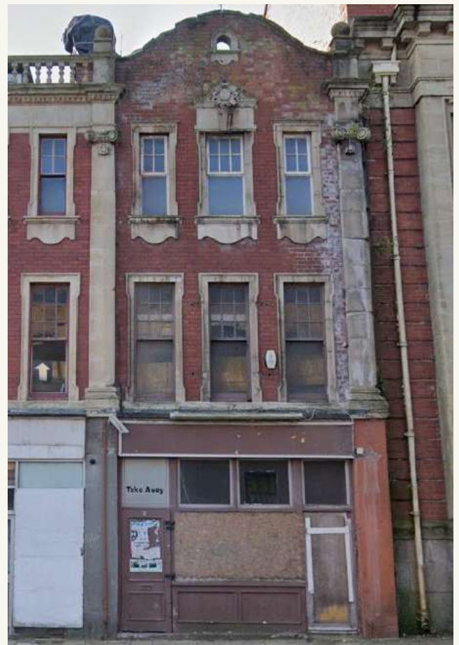
Figure 3.7 – Front elevation of no.10, prior to recent repair works (March to June 2021).
