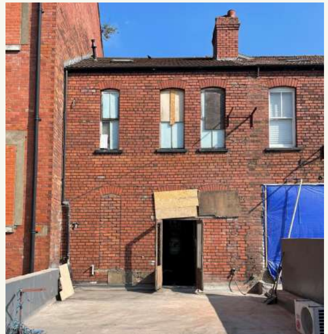
Figure 3.11 – Rear elevation of no.10, photo taken during recent repair works
