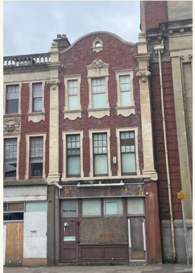
Figure 3.9: Exterior of the front facade July 2022
