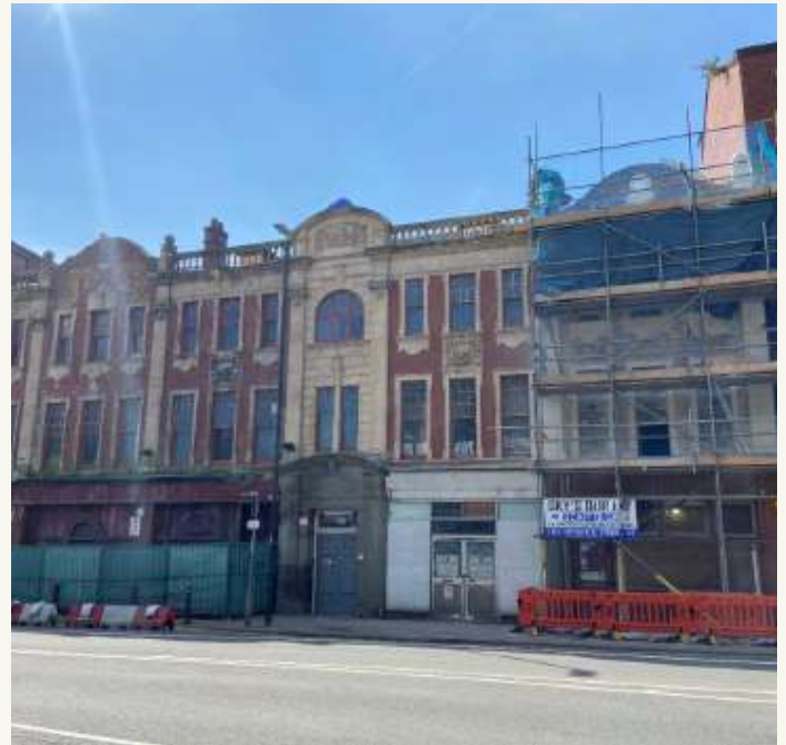
Figure 5.1 – Nos. 10-18 Clarence Place (the application site is scaffolded)
