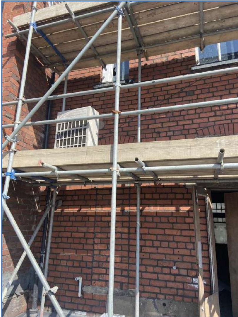
Images 11 and 12 – Rear elevation of no.10 Clarence Place (prior to repair works to masonry).
