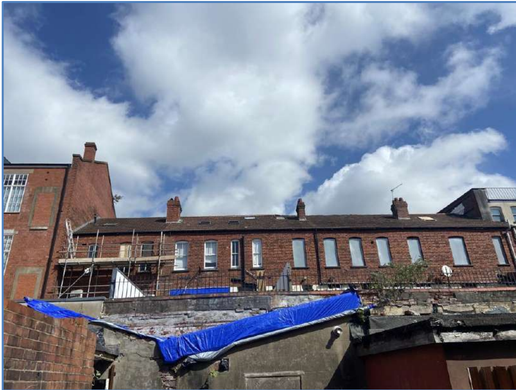
Images 7 and 8 – Rear elevation of no.10 Clarence Place (prior to repair works to masonry).
