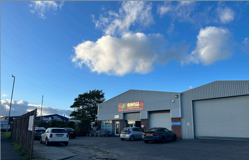
Figure 11 - Maesglas Industrial Estate
