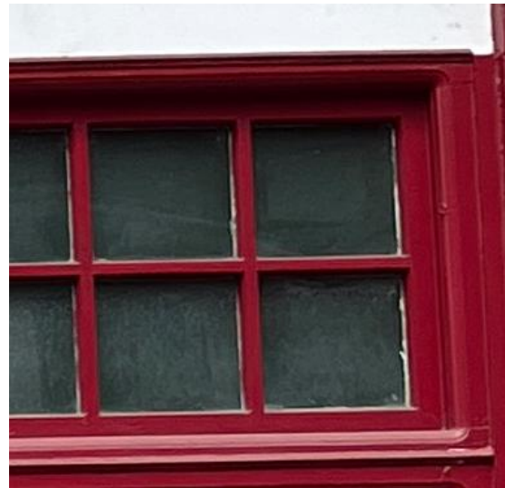
Existing fan Light small single pane glazing to shopfrontage, painted finish, within hardwood simple square framing
