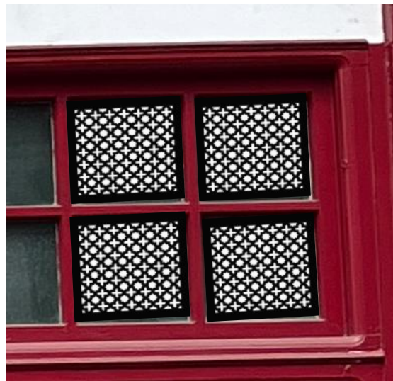
Proposed 4 panes glazing removal and kept on site. Salvaged cast iron Victorian vent grilles fitted in place.
