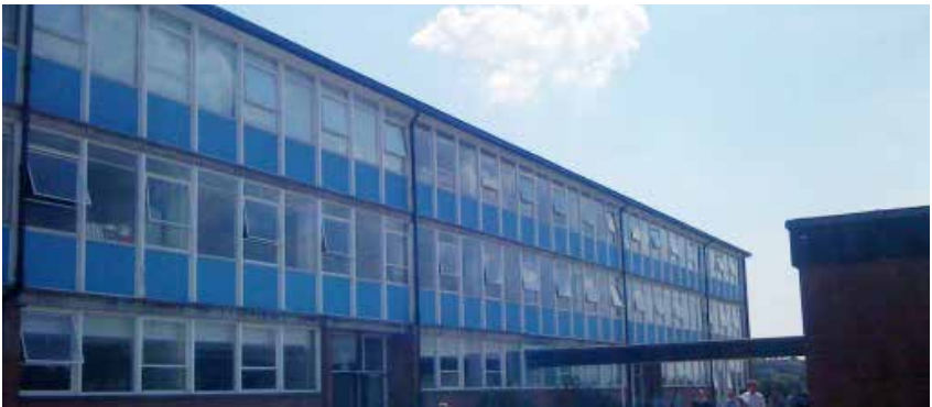
Below: The sixth form block echoes the single storey J & F blocks, although with taller proportions. It shows alternating vertical strips of pale brickwork, with individual windows and panels.
