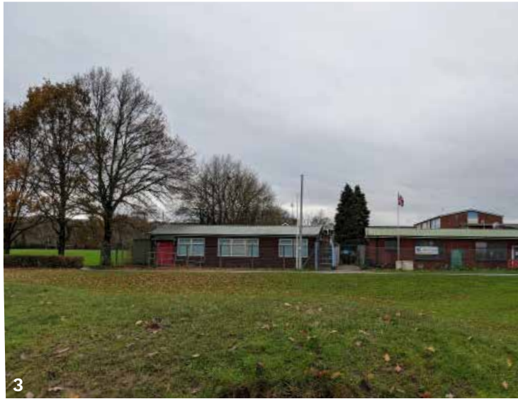
View 3: View of existing school site from the southern stretch of Cold Bath Road, part of CCA. The image begins to show the level of transparency associated with the site's south-eastern tree line border during winter months.
