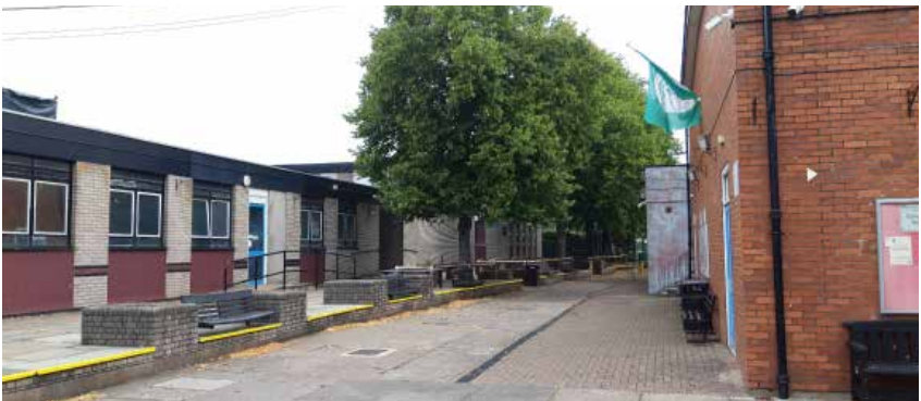
Below Right: The majority of ABC block is curtain walling, thought to be the original, with a red brick plinth and ends. The corner of J block can just be seen, with the service 'bridge' connecting them.
