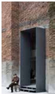
EXTENDED WINDOW FRAME REVEALS Reduces use of brick in reveals, keeping material palette simple.
