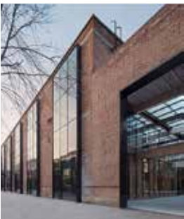
EXTENDED WINDOW FRAME REVEALS Reduces use of brick in reveals, keeping material palette simple.
