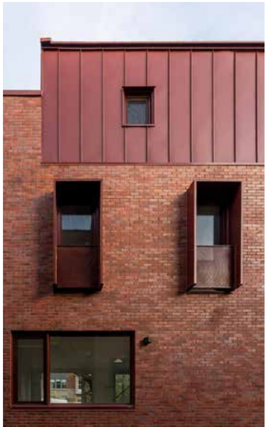
EXTENDED WINDOW FRAME REVEALS Reduces use of brick in reveals, keeping material palette simple.
