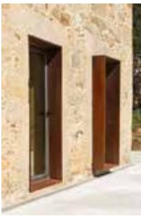
EXTENDED WINDOW FRAME REVEALS Reduces use of brick in reveals, keeping material palette simple.
