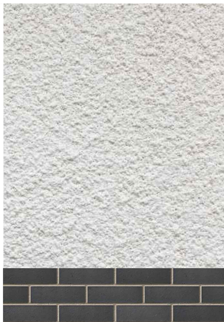
Image 06: staffordshire blue engineering brick plinth
