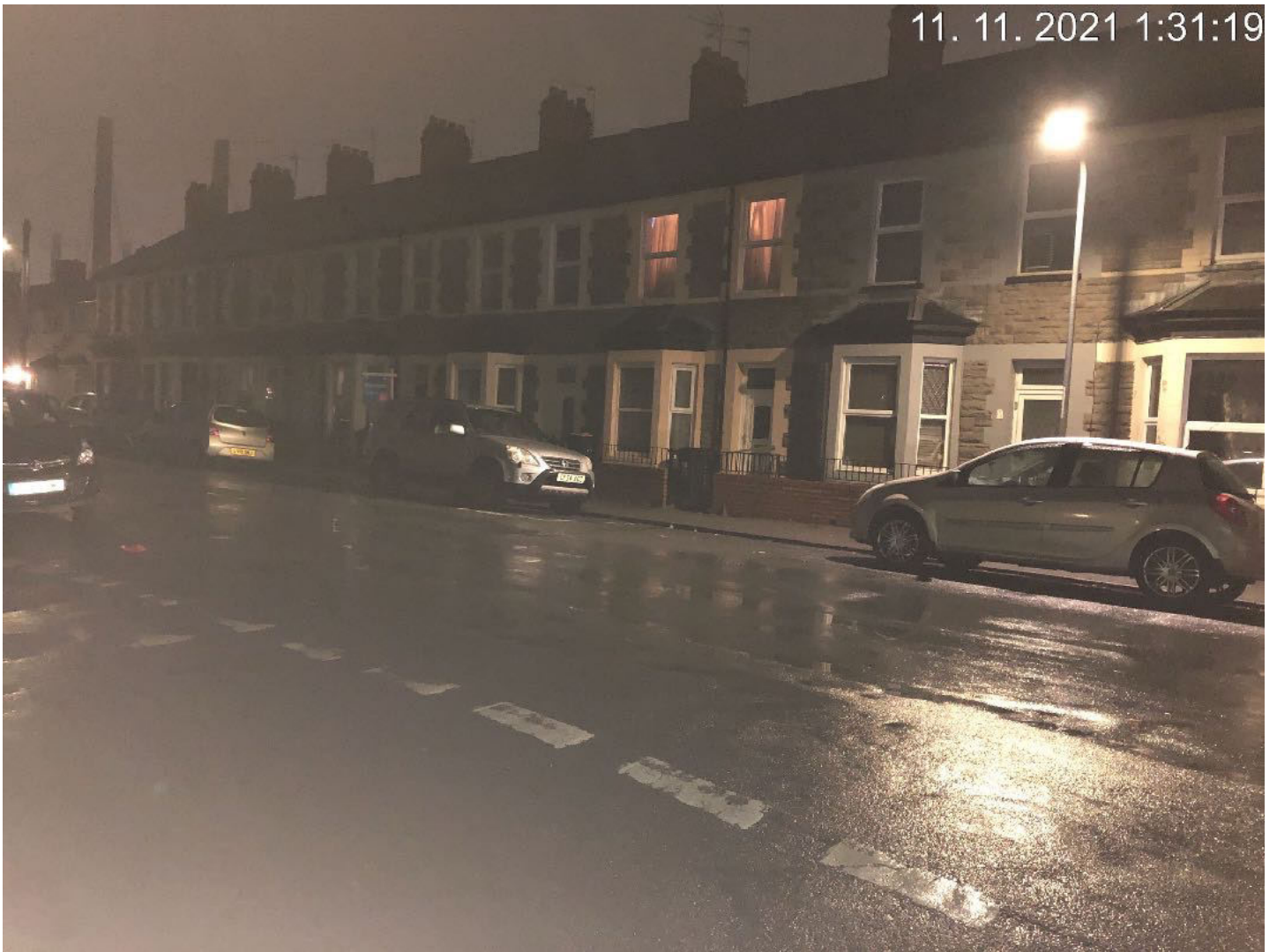
11-Nov-21: Coverack Road facing South-West
