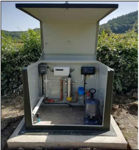
Typical insulated, lockable glass reinforced plastic Borehole cabinet
