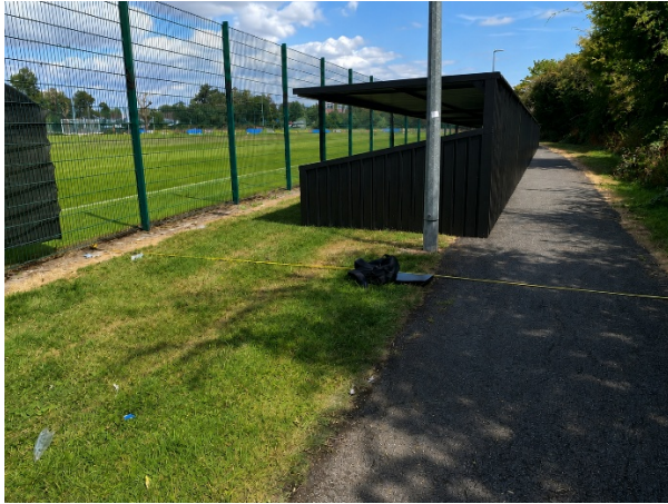
Figure 8 Photograph of path from Velodrome end, with spectator stand added to 4.1m from fence
