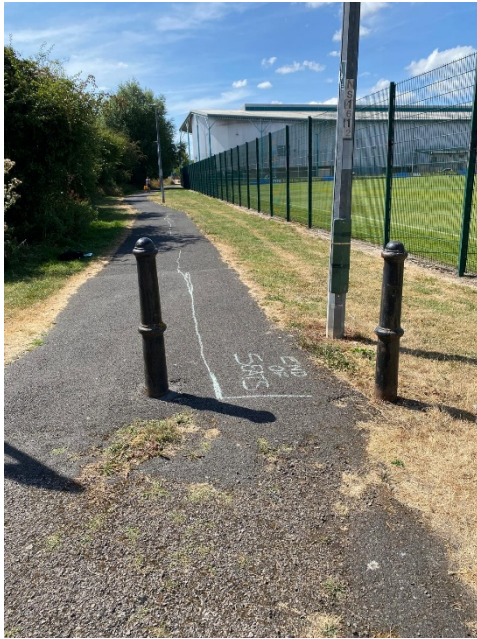
Figure 5 Straight line drawn 4.1m from existing fence showing reed vegetation on left
