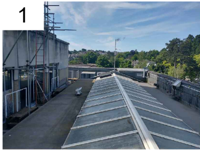
Existing roof lantern to be cleaned and retained
