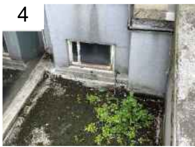
Redundant low-level window to be removed and infilled with brickwork
