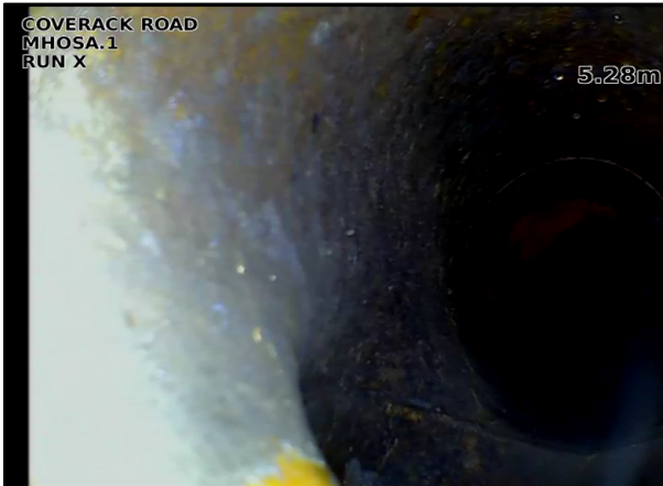
Photo: 8_8_147_A.jpg, 00:01:14 5.28m, Finish node type, manhole reference number: MH01 A
