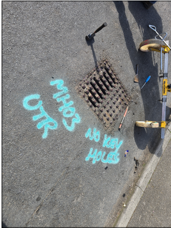
Photo: 20250401_114610.jpg 0m, Start node type, manhole, reference number : MH03 UTR
