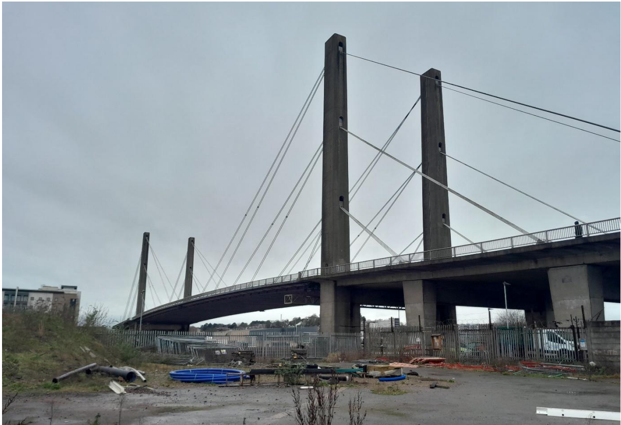
Image EDP A1.2: North-west facing view of the Site ground conditions from the north-east corner of the Site. Image also illustrates the proximity of the Site to the Grade II* George Street Bridge (25847).
