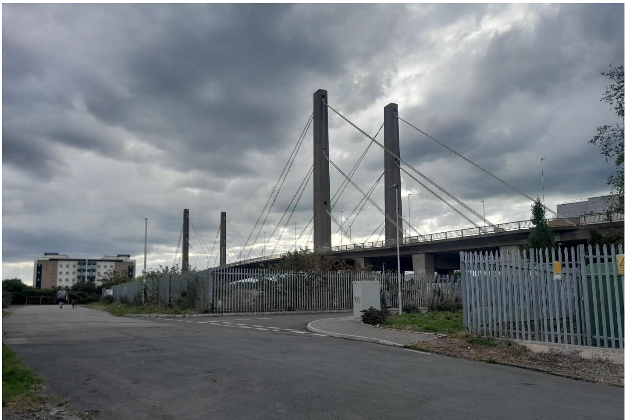
Image EDP A1.11: West facing view from the southern end of Coverack Road adjacent to the Site. View towards the Grade II* listed George Street Bridge (25847).
