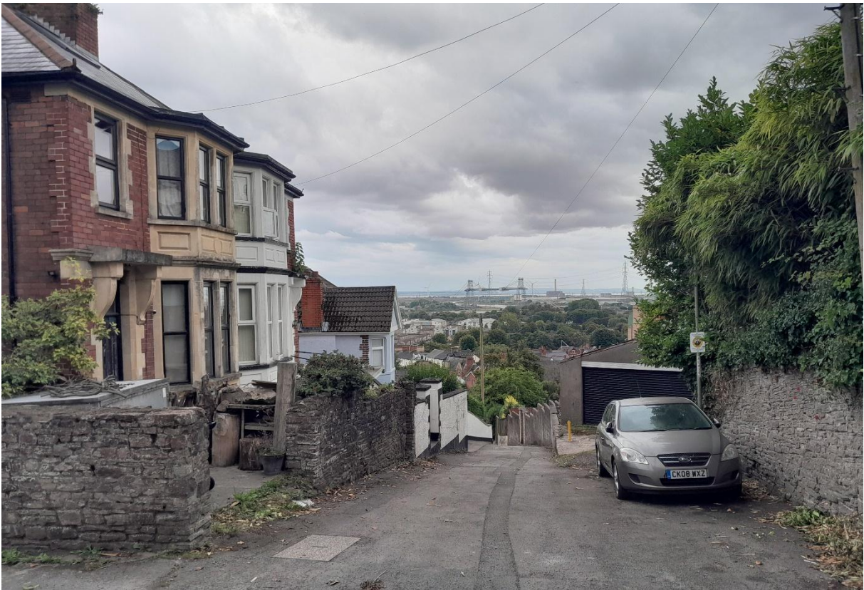
Image EDP A1.21: South-east facing view from Vicarage Hill towards the Grade I listed Transporter Bridge including E and W anchor chambers (3076).
