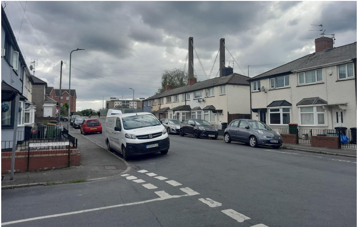
Image EDP A1.10: West facing view from the corner of Coverack Road and Feering Street towards the Grade II* listed George Street Bridge (25847).
