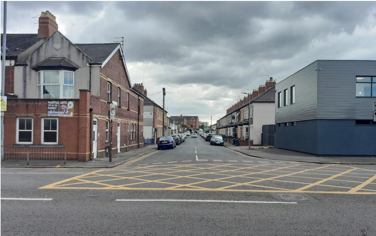
Image EDP A1.8: South-west facing view from Corporation Road down Coverack Road. Image looking down Coverack Road towards the Site and the Grade II* listed George Street Bridge (25847), beyond the terraced row of housing on the right side of the street. As shown neither are visible from the junction between Coverack Road and Corporation Road.
