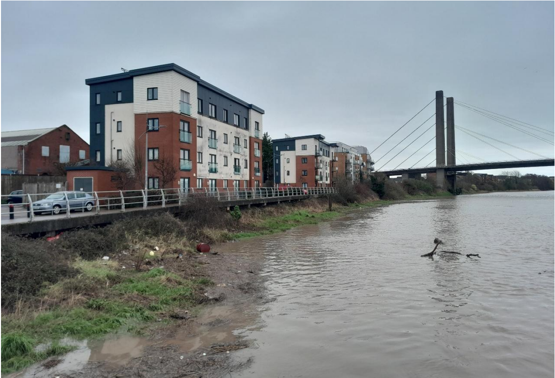
Image EDP A3.2: View looking along the eastern riverside illustrating its present character populated by modern residential buildings.
