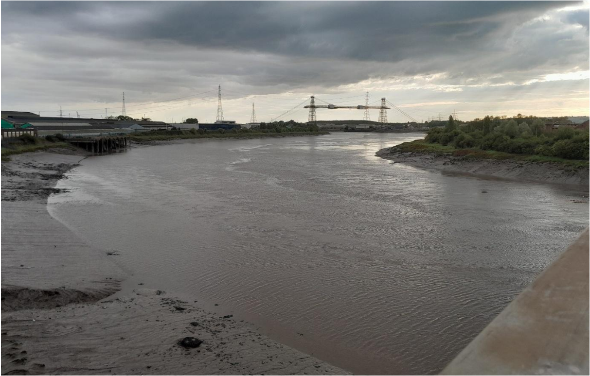
Image EDP A1.20: South-west facing view from 2004 built City Bridge towards the Grade I listed Transporter Bridge including E and W anchor chambers (3076).
