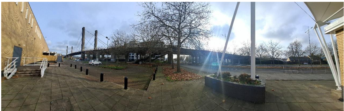
Image EDP A3.15: Panorama of the view in Image A3.14 , illustrating the full extent of the bridge that is visible in this view.
