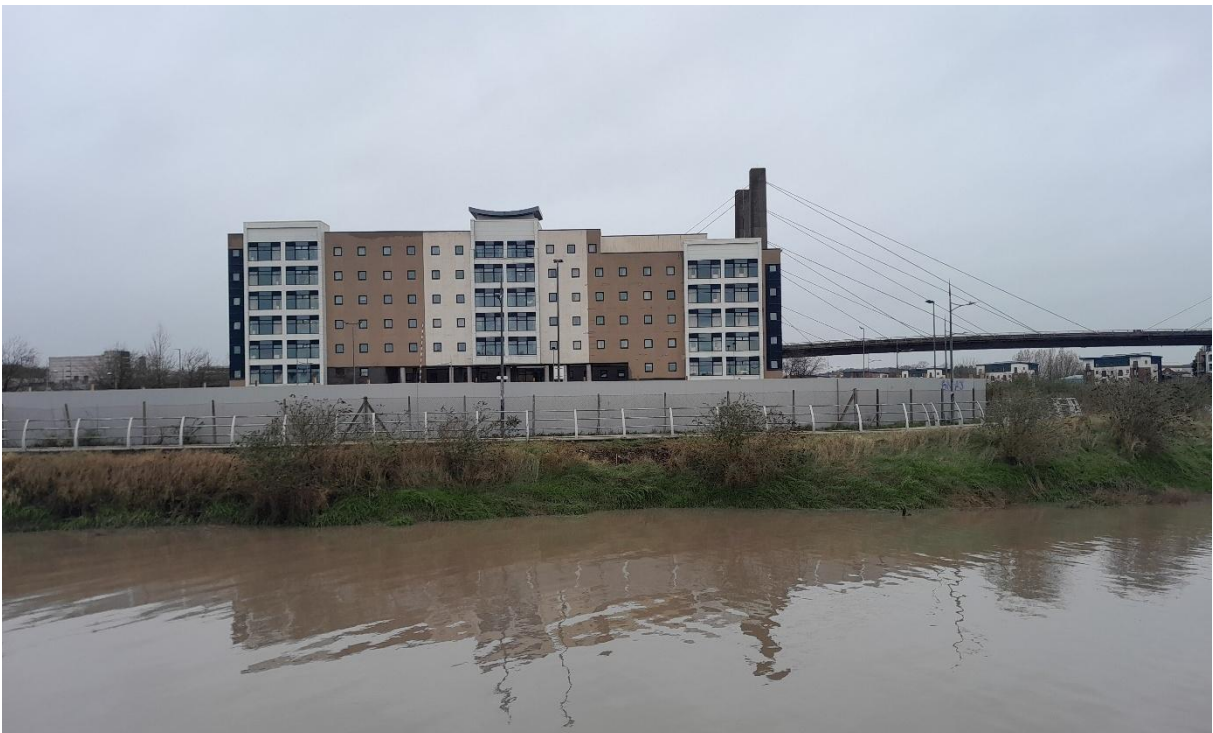
Image EDP A1.19: North facing view of the seven-storey Newport Student Village flat block development on the west side of the River Usk. Image to show the scale, massing and height of the flat block in relation to the adjacent Grade II* listed George Street Bridge (25847).
