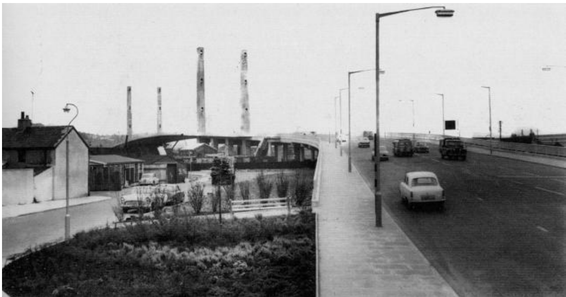
Image EDP A3.13: Historic photograph looking towards the site from the west to illustrate how the bridge's setting has changed.
