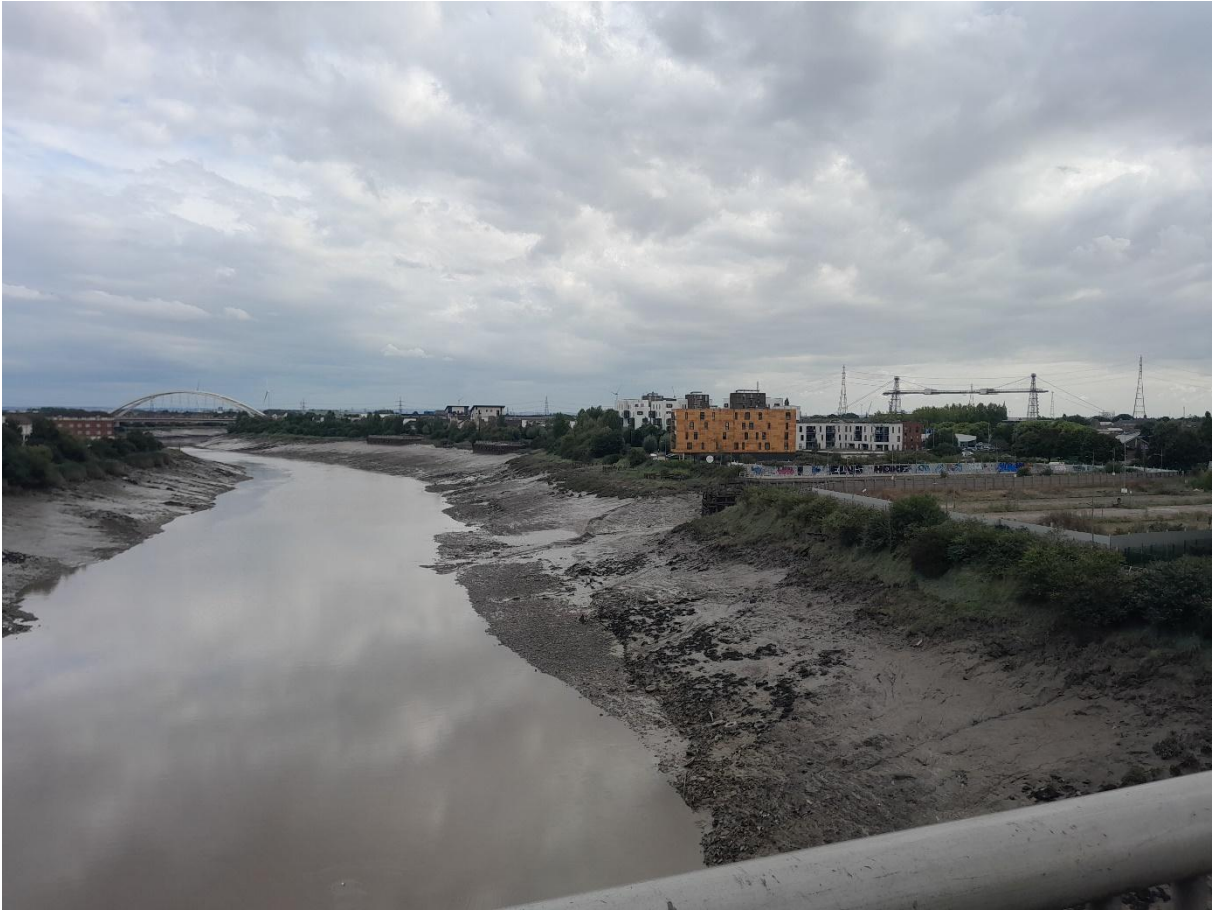
Image EDP A1.24: South facing view towards the Grade I listed Transporter Bridge including E and W anchor chambers (3076) from the centre of the Grade II* George Street Bridge (25847). Image to illustrate how clear, full views of the Transporter Bridge from along the centre of the George Street Bridge will be unaffected by development within the Site.
