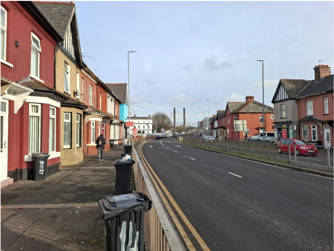
Image EDP A3.10: View towards the bridge from George Street showing how some older buildings are retained.
