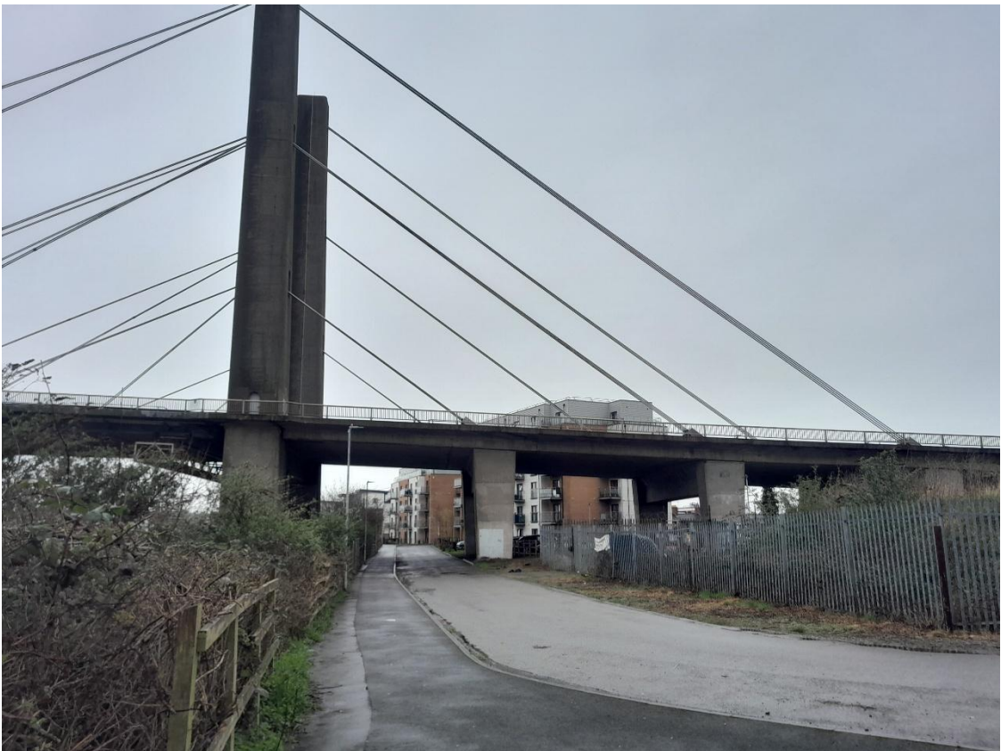
Image EDP A3.3: View looking north to the bridge from the western end of Coverack Road. The disused, derelict land to the right is the site.
