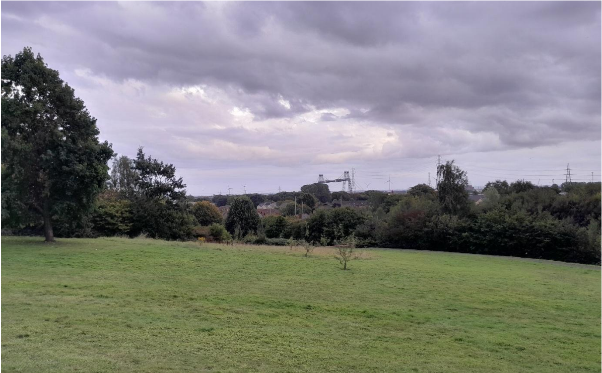
Image EDP A1.22: South-east facing view from Belle Vue Park towards the Grade I listed Transporter Bridge including E and W anchor chambers (3076).
