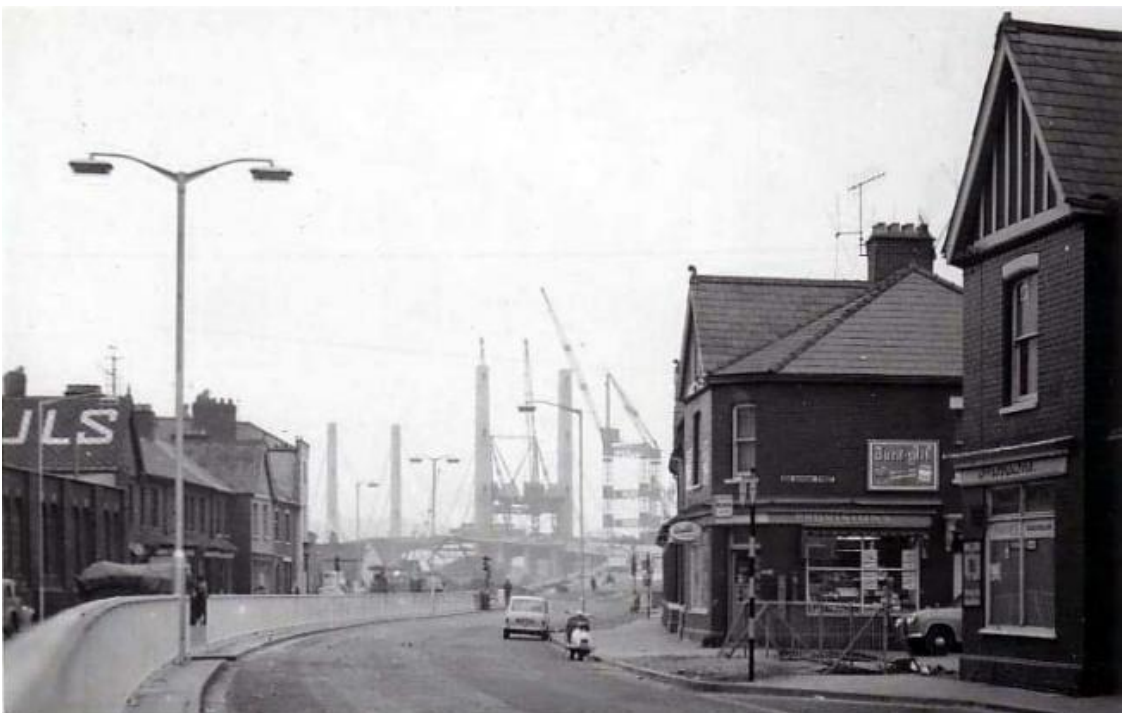
Image EDP A3.11: Historic photograph looking towards the site from George Street to illustrate how the bridge's setting has changed.
