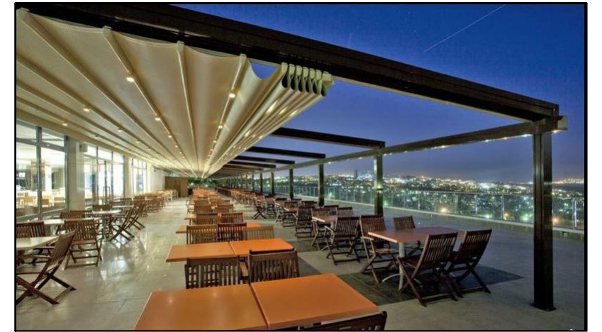
RETRACTABLE TENSILE STRUCTURE
