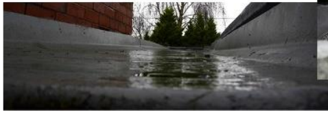
Building One - Rubber membrane
