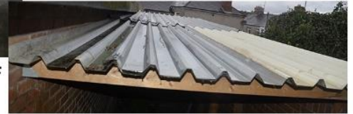
Building Three - Corrugated steel roof
