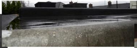
Building Two - Concrete roof
