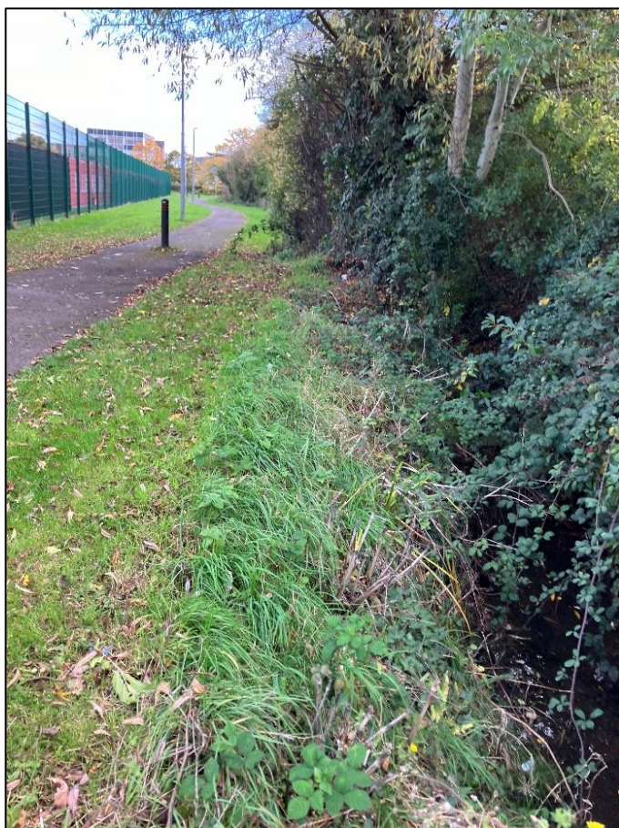
Figure 7-A: Drainage ditch adjacent the southern boundary of the existing grassed pitch
