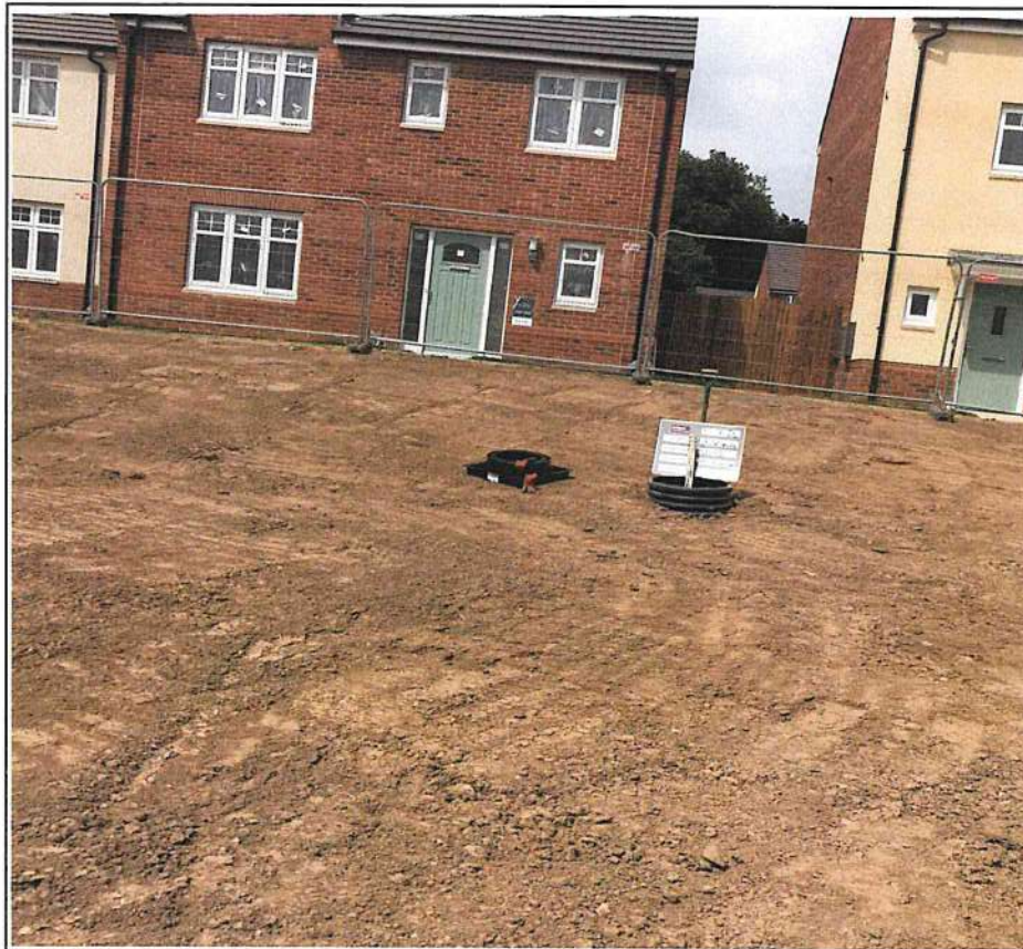
POS Area (Adjacent to Plot 423) A Depth Check
