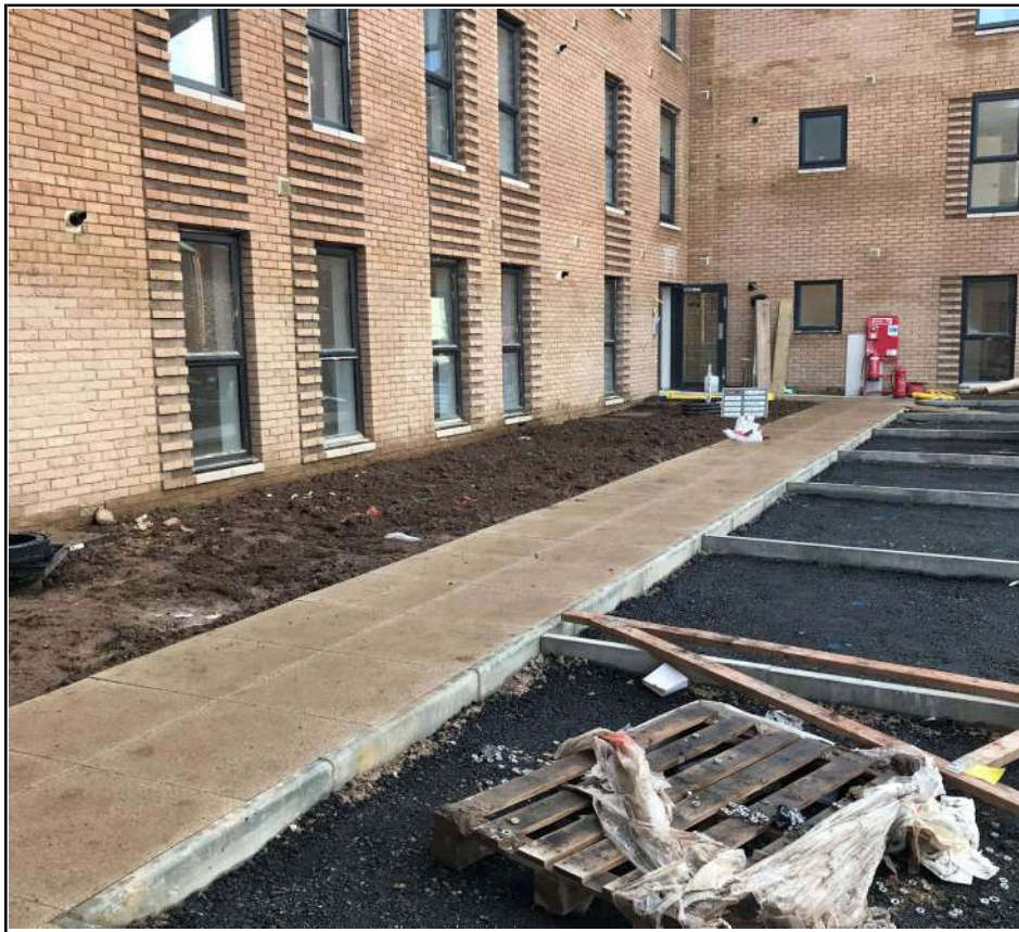
Block P Infilled landscaping Main Entrance
