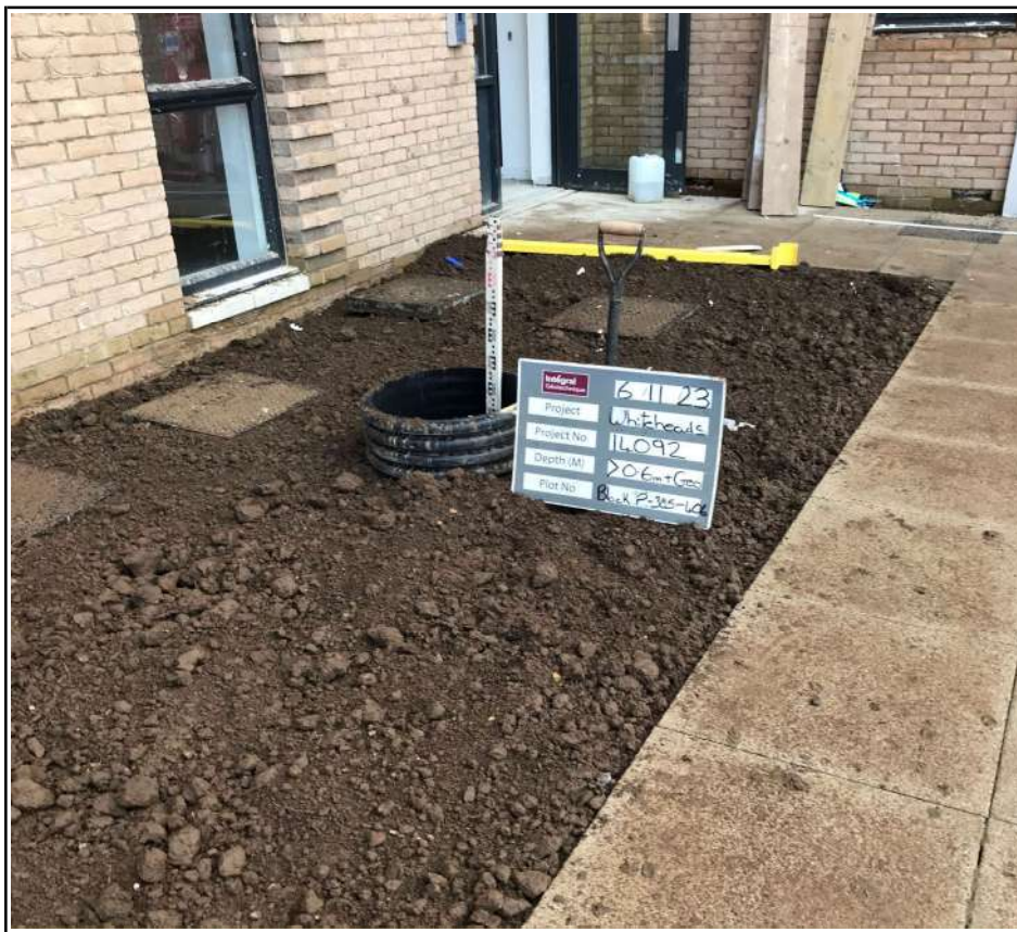
Block P Capping Depth Validation Check
