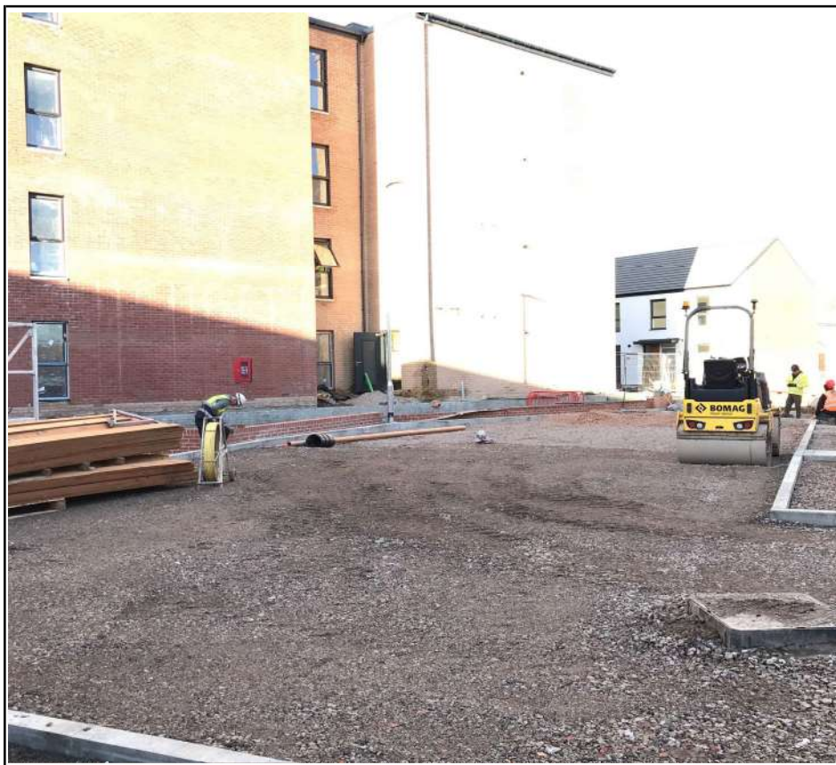
Block P Carpark Area Under Construction
