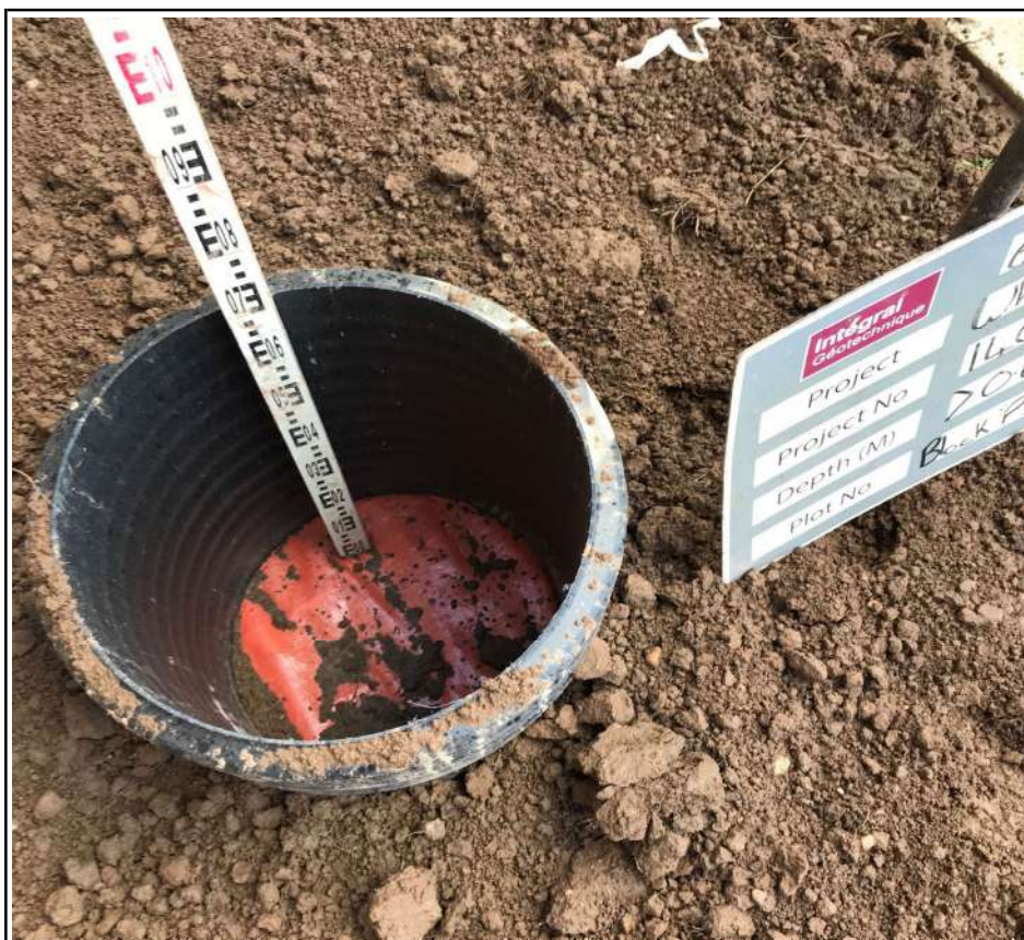
Block P Membrane Placement Check
