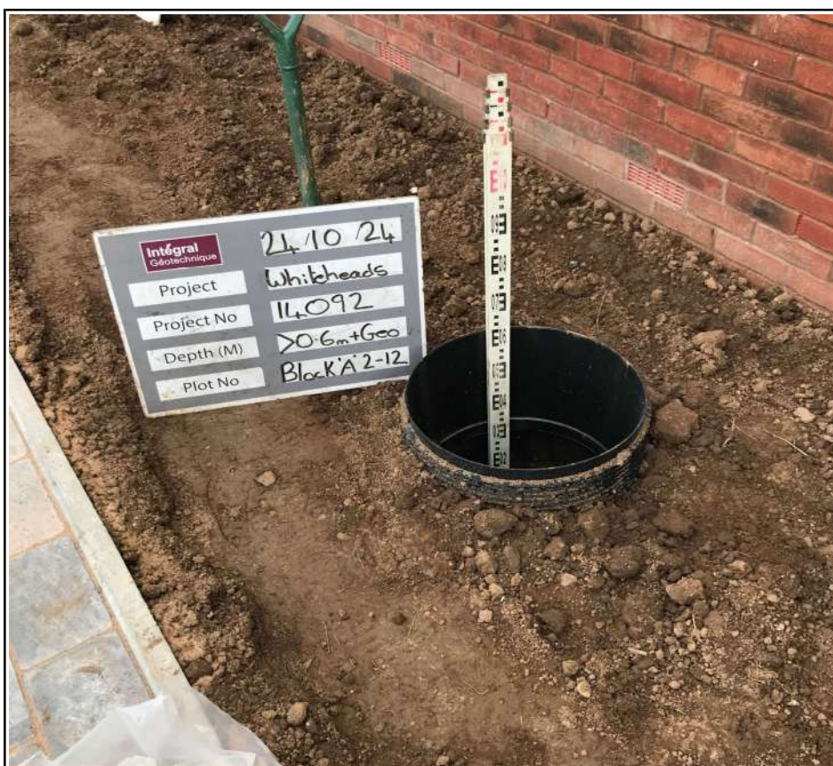
Block A Capping Depth Check
