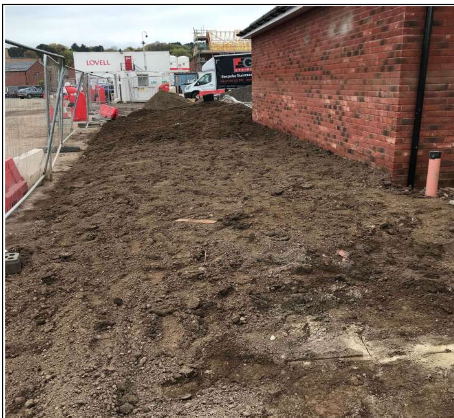
Block A Southern Flank Soil Infill
