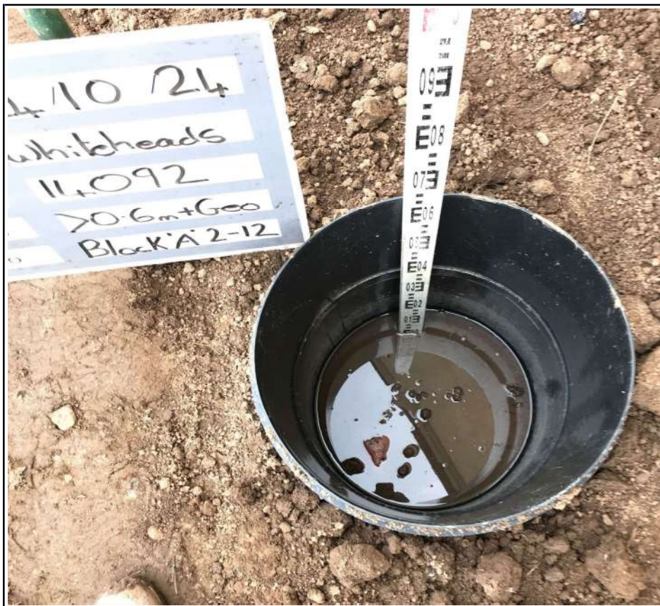
Block A Membrane Placement
