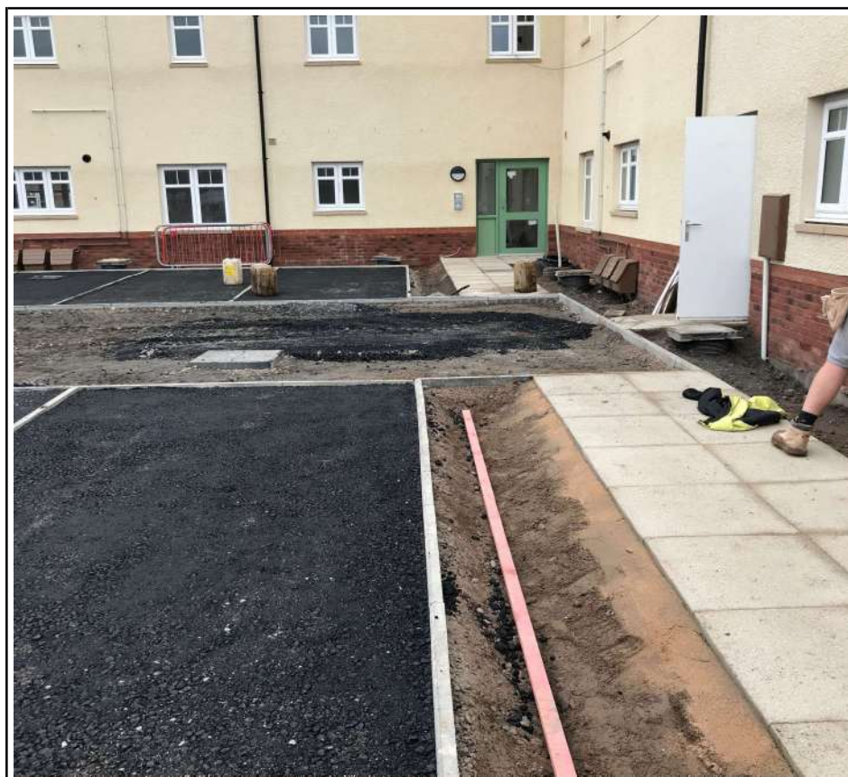
Block A Rear of Apartment Block to Carpark Finish
