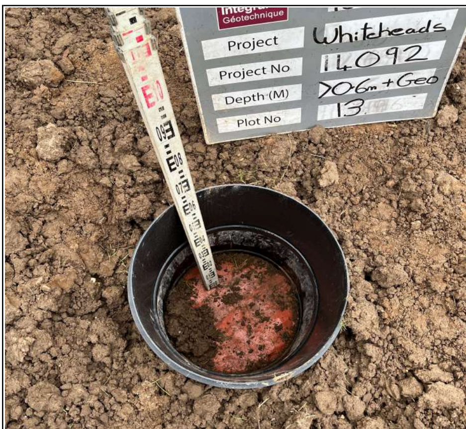
Plot 13 Trial Pit Excavation (Topsoil Only) Membrane Placement
