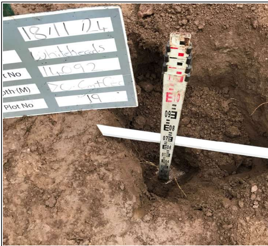
Plot 19 Membrane Placement
