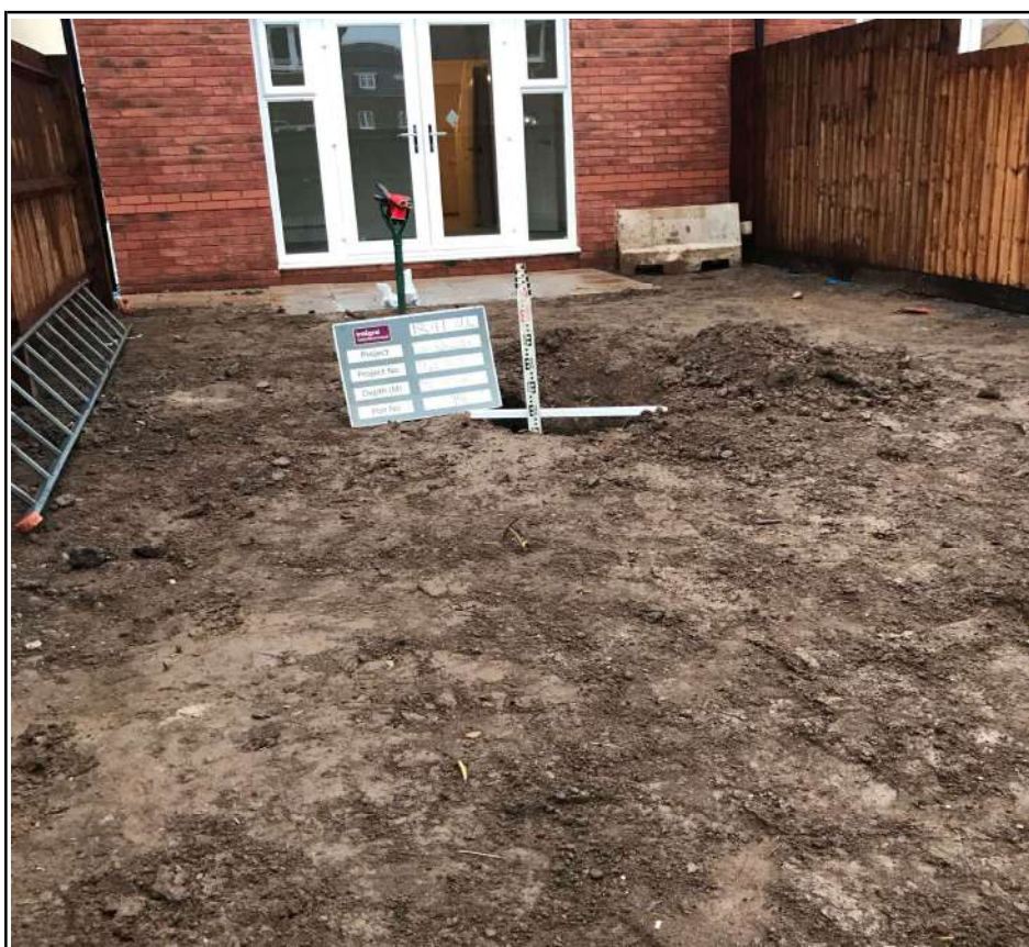
Plot 19 Capping Depth Check
