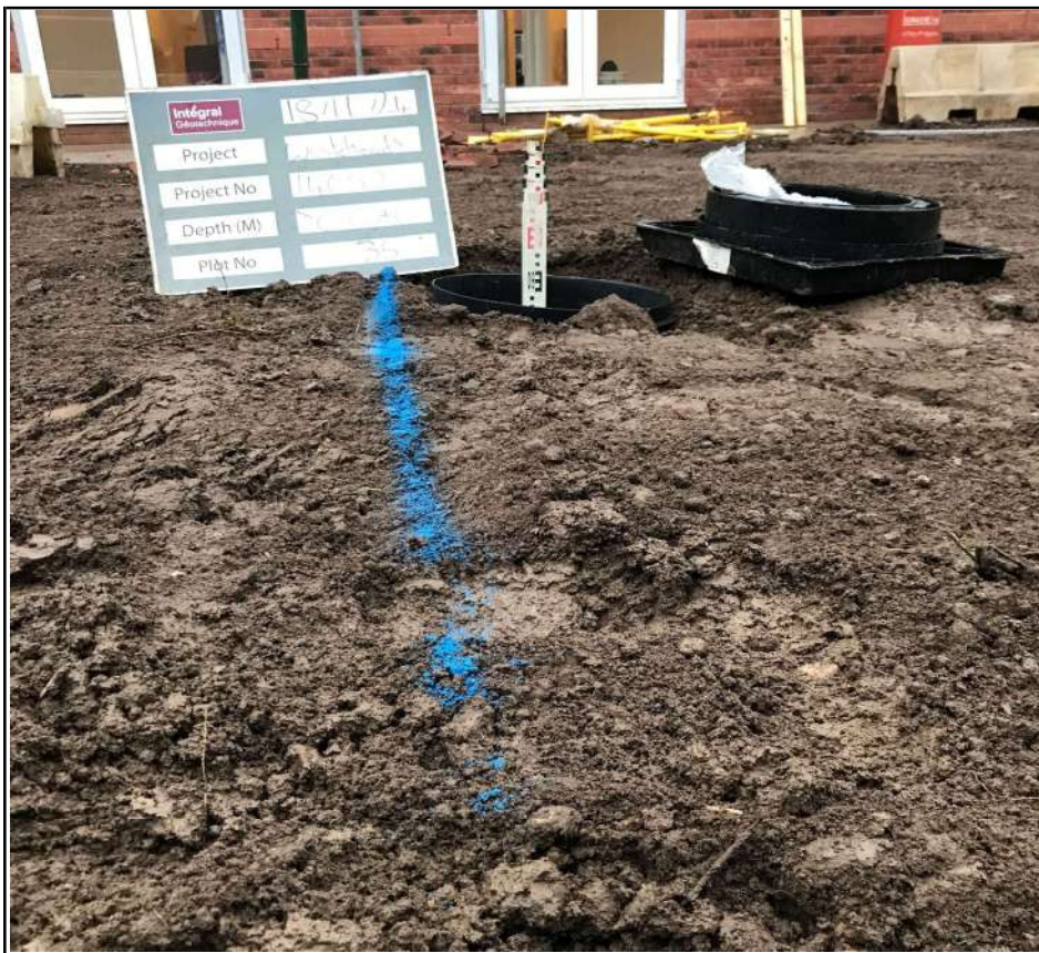
Plot 35 Capping depth Check
