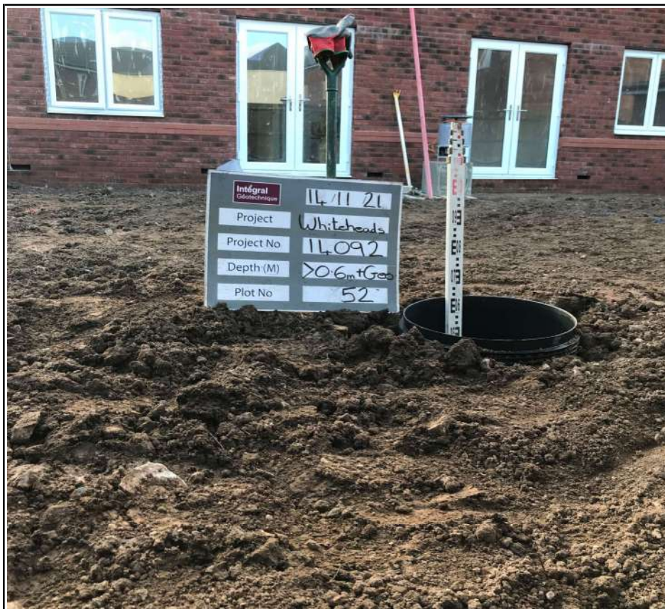
Plot 52 Capping Depth Check
