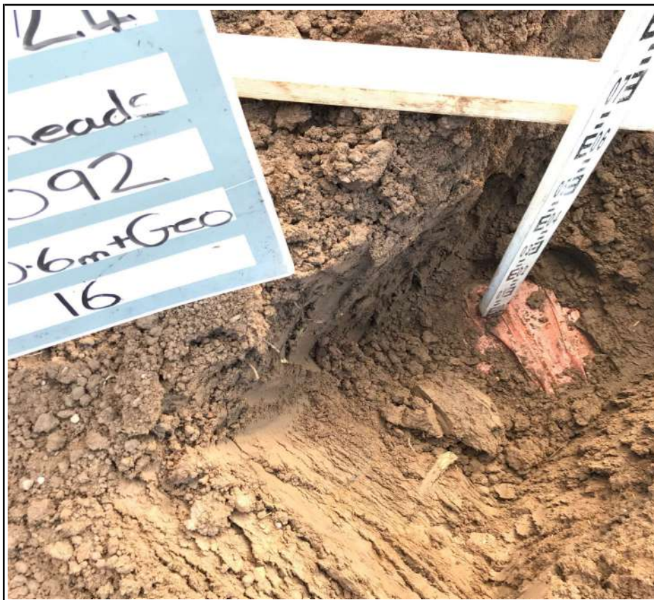
Plot 16 Membrane Placement
