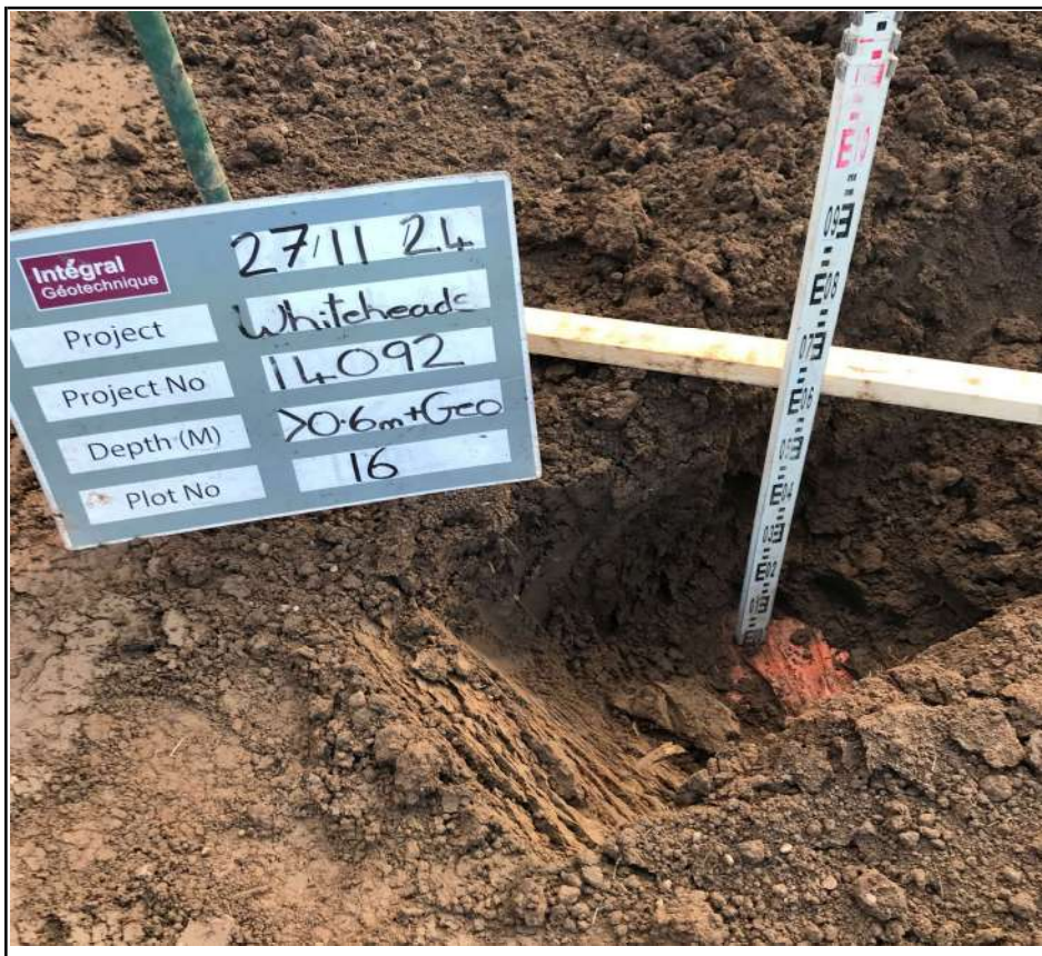
Plot 16 Trial Pit Excavation Profile (Topsoil Only)
