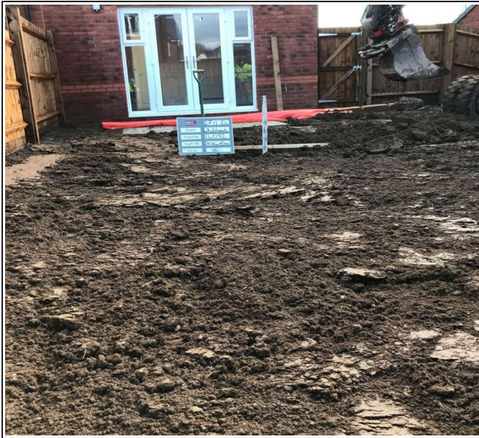
Plot 16 Capping Depth Check
