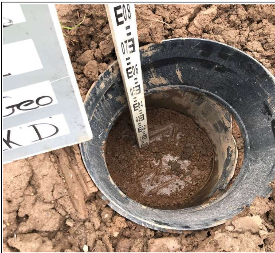
Block D Membrane Placement
