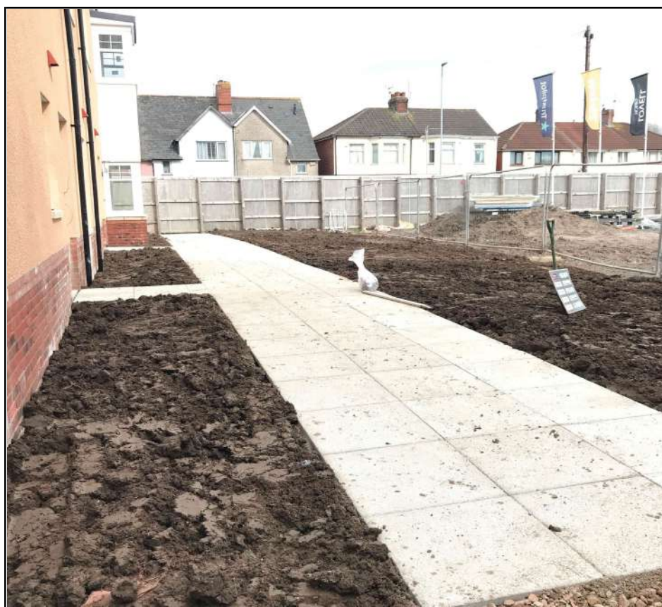
Block D Infilled Landscaped Area
