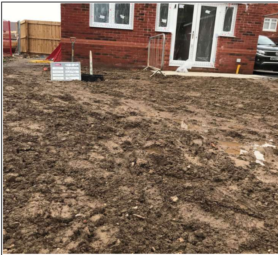
Plot 34 Capping Depth Check
