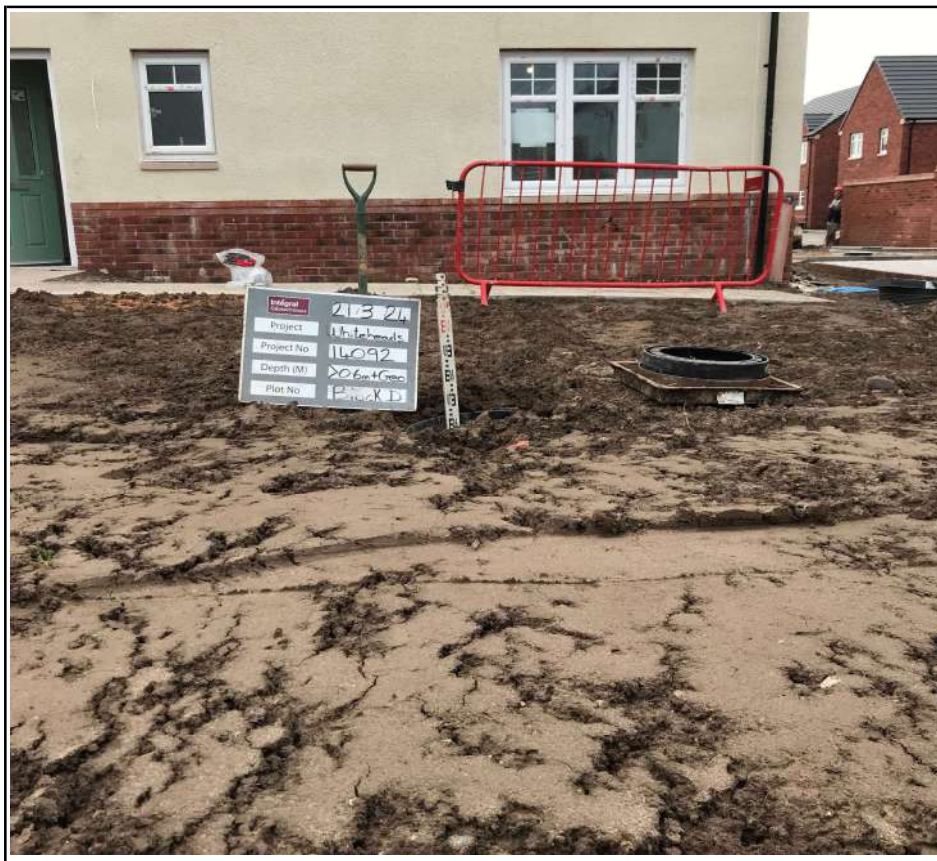
Block D Capping Depth Check
