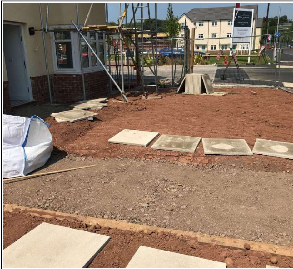
Block E plots 73 to 81 Area to Main Entrance
