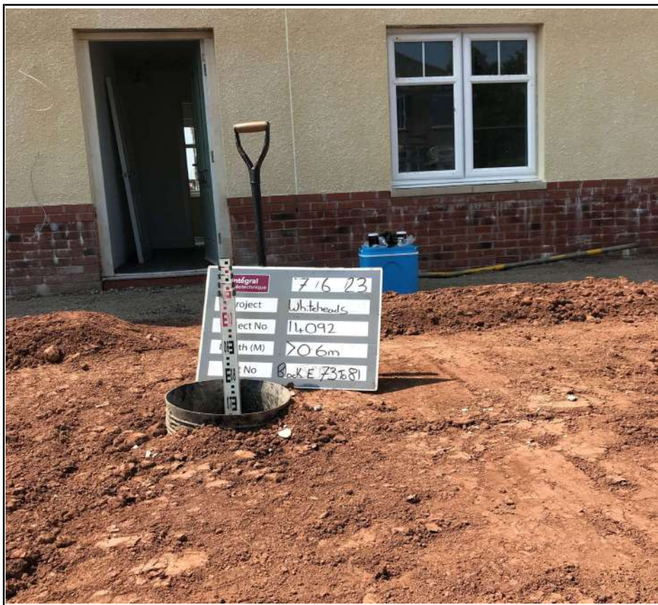
Block E Plots 73 to 81 Capping Depth Check
